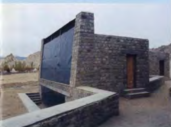
11. Completed solar-assisted VIP latrine.
