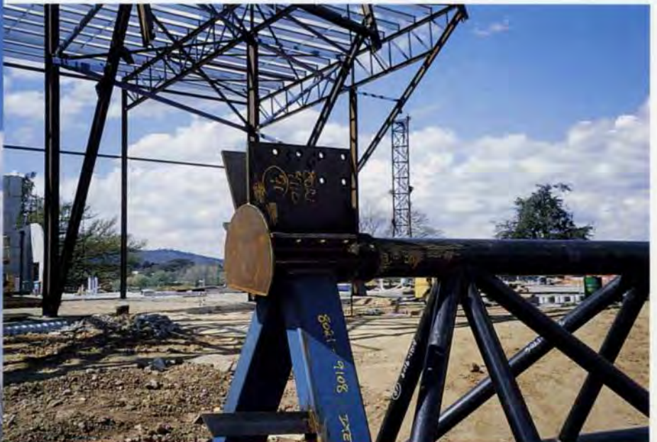
7 above: Foreground: Temporary Gallery structure (in unpainted steelwork, for cost saving) awaiting erection; in the background is the first Main Hall tower.
