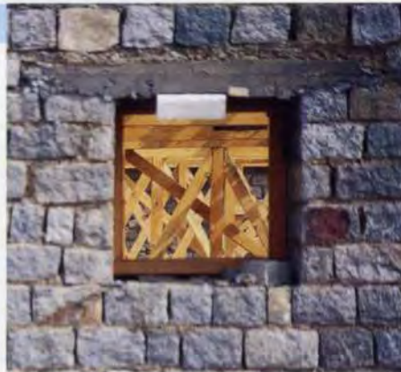
18. Local stone and timber: appropriate materials.
