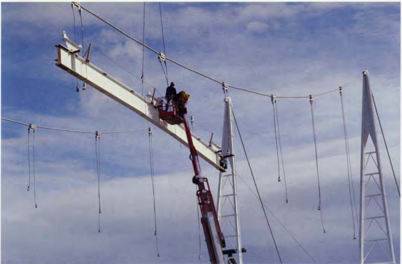
4. Hanging roof beam from the cable.
