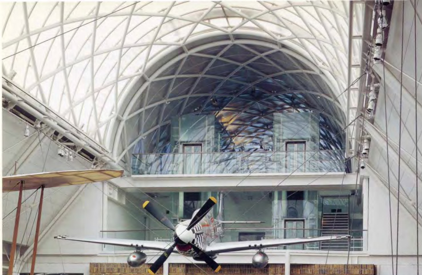
10. Close-up of main staircase at the upper levels, showing the link between the Stage 1 and Stage 3 barrel vaults.
