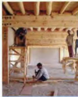
5. Construction in progress.
