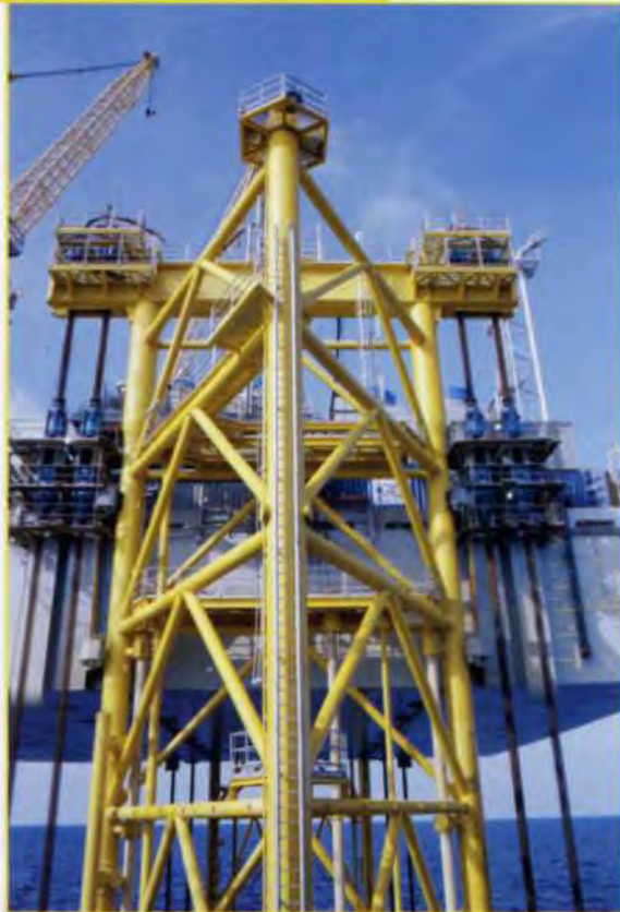
8. Deck raised to final elevation.
