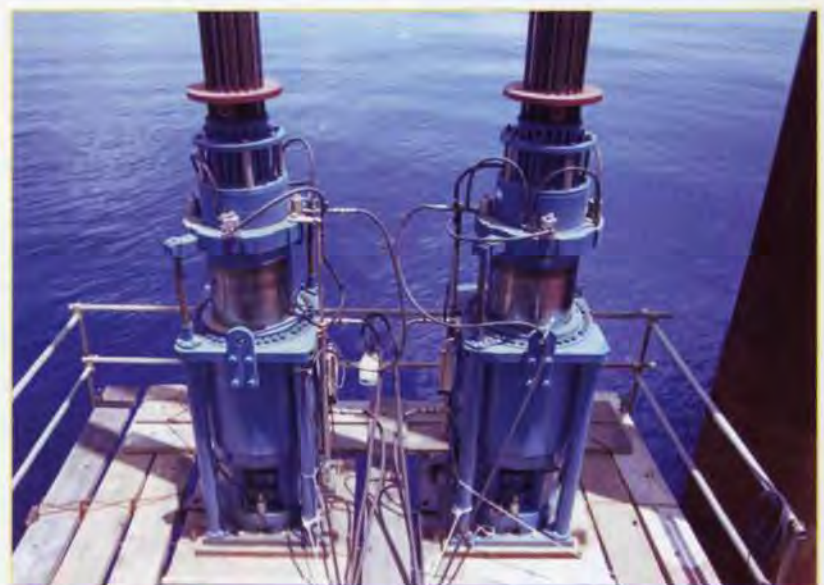
6. Base lowering jacks.
