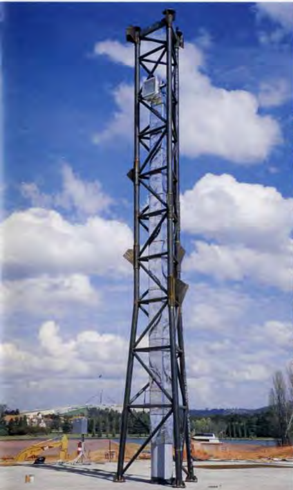
7 above: Foreground: Temporary Gallery structure (in unpainted steelwork, for cost saving) awaiting erection; in the background is the first Main Hall tower.
