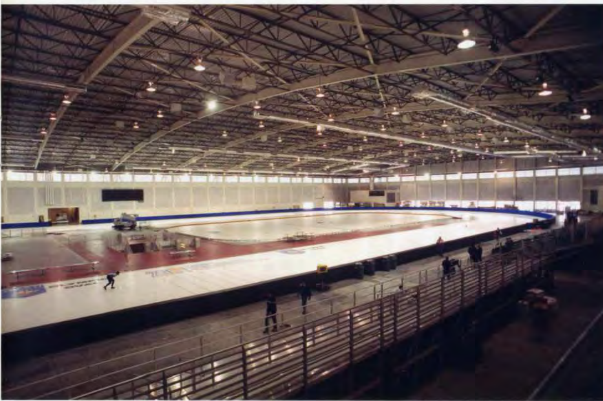
14. Interior artificially lit, showing shaded clerestory windows admitting daylight.
