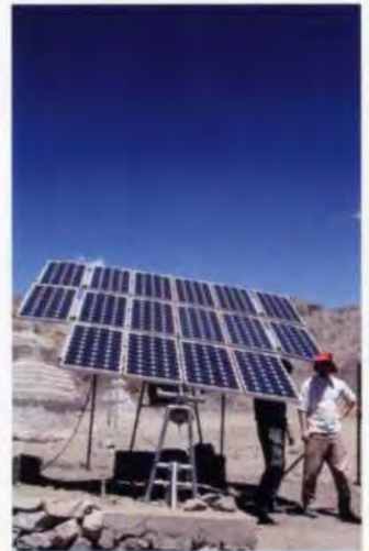
7. Solar panels power water pump.
