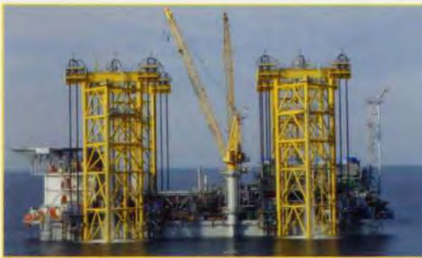
7. Pumping during installation of skirted base.
