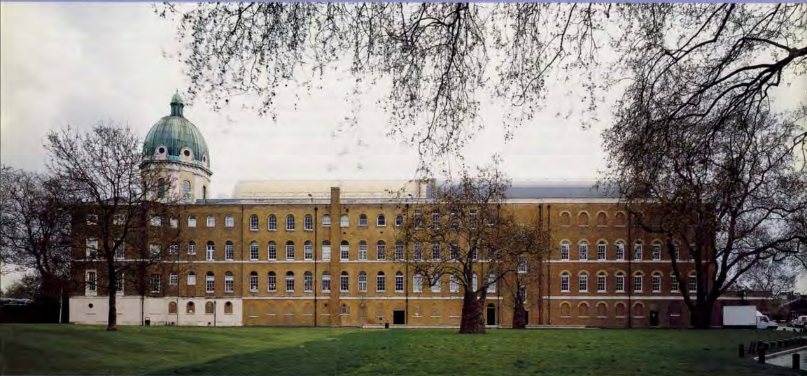
1. West façade of completed building.
