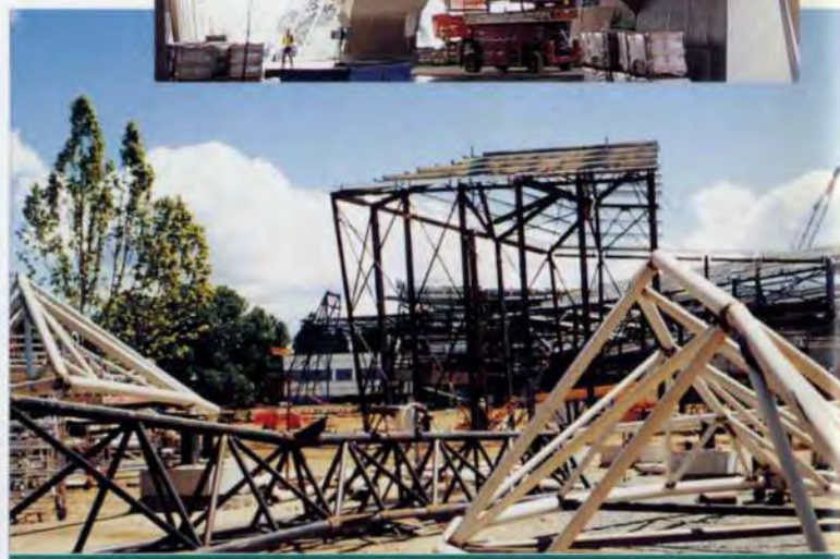
18. Skylight fabrication, with Gallery of the First Australian steelwork in background.
