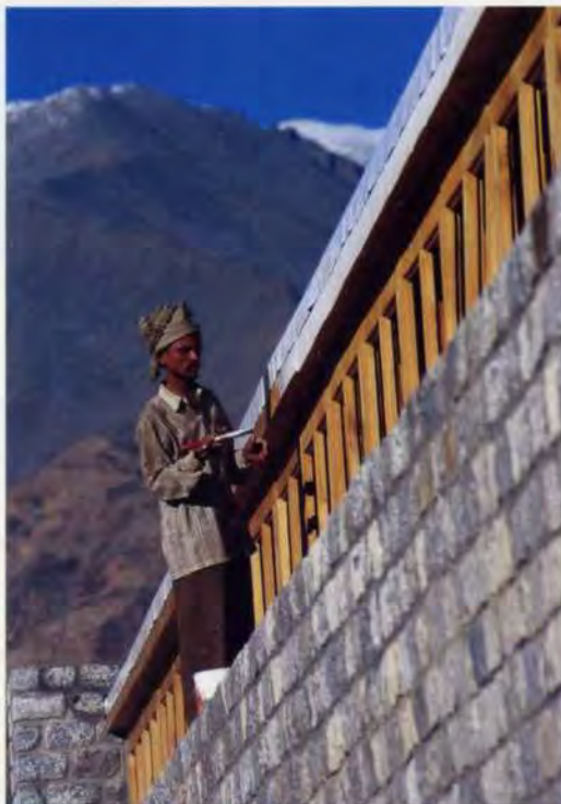
17. Painting the roof eave above timber-framed windows.
