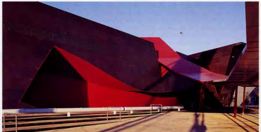
14. 'Loop' canopy and main entrance tunnel.
