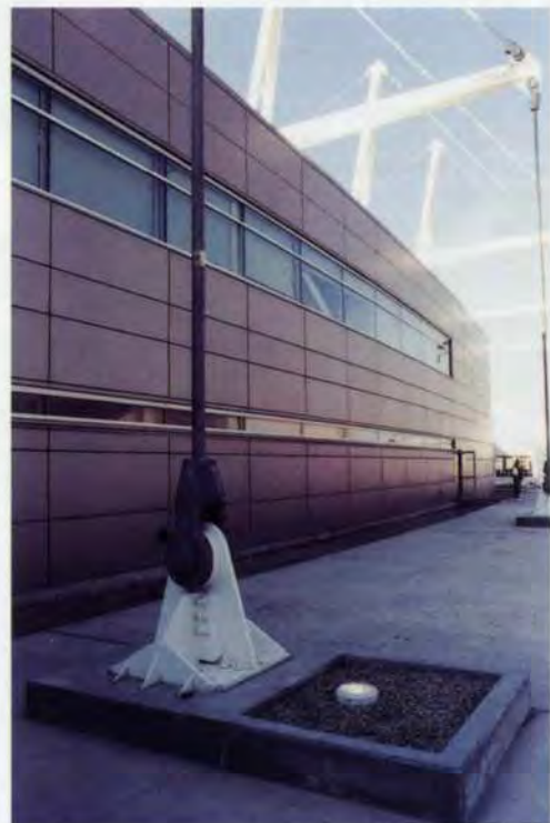
8. Tie down connection detail.
