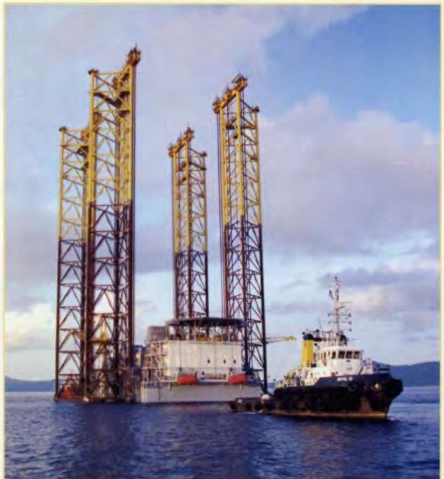
1. Platform ready for wet tow.
