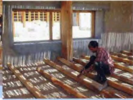
6. Laying the floor.
