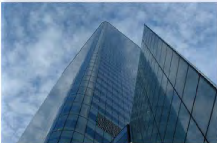
12. View up the completed HSBC tower.
