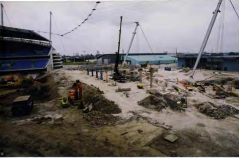
5. left: Removal of temporary seating, 2 September 2002.
