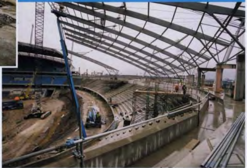
6. below: Progress on the North Stand, 21 January 2003.
