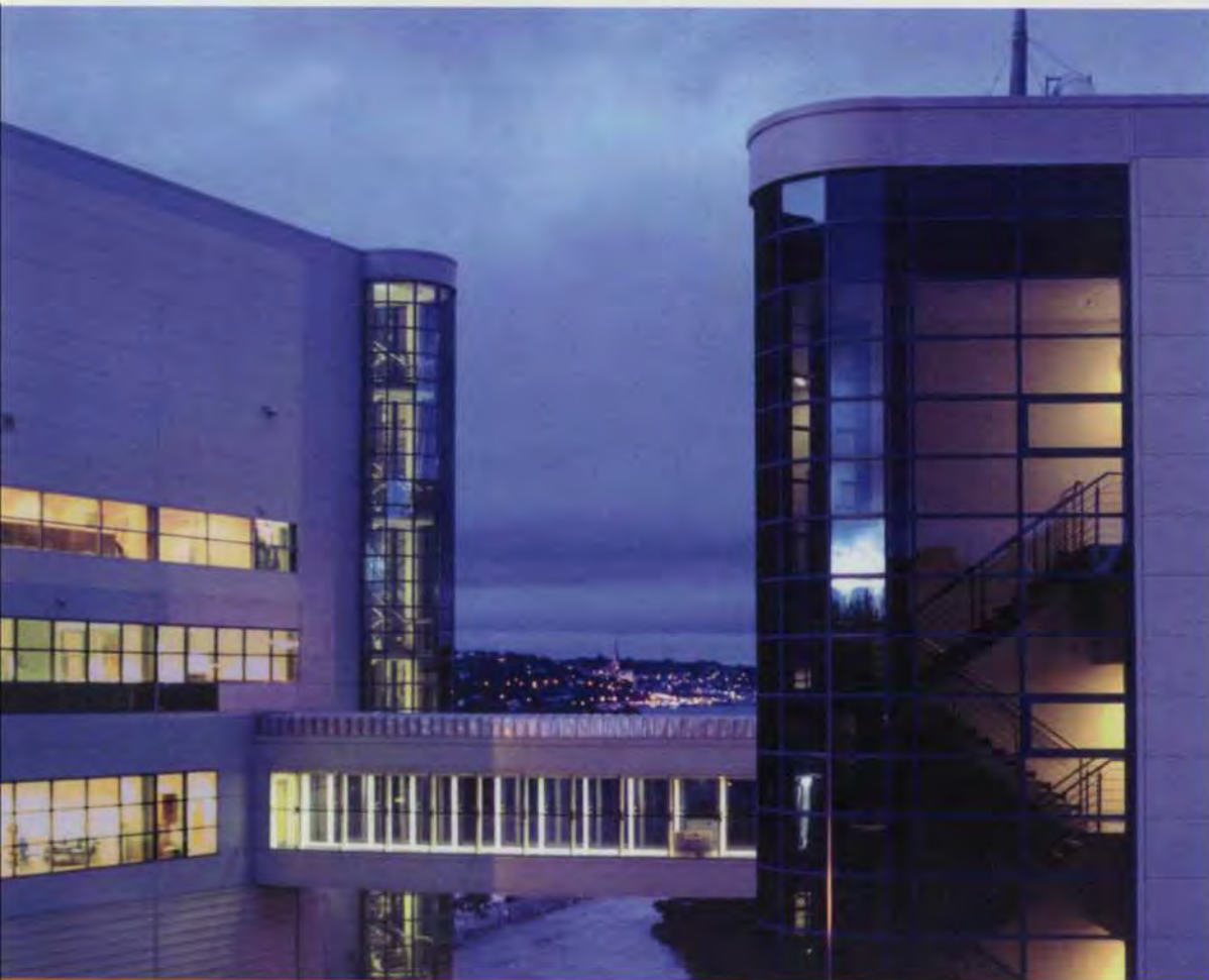
21. Evening view of the link bridge between the production building and the finished goods building.
