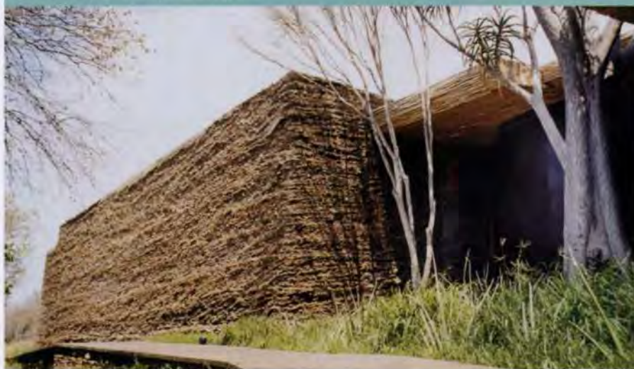
11. The completed compacted earth wall.
