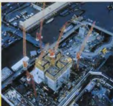
11a-d: Self-climbing core formwork construction sequence.
