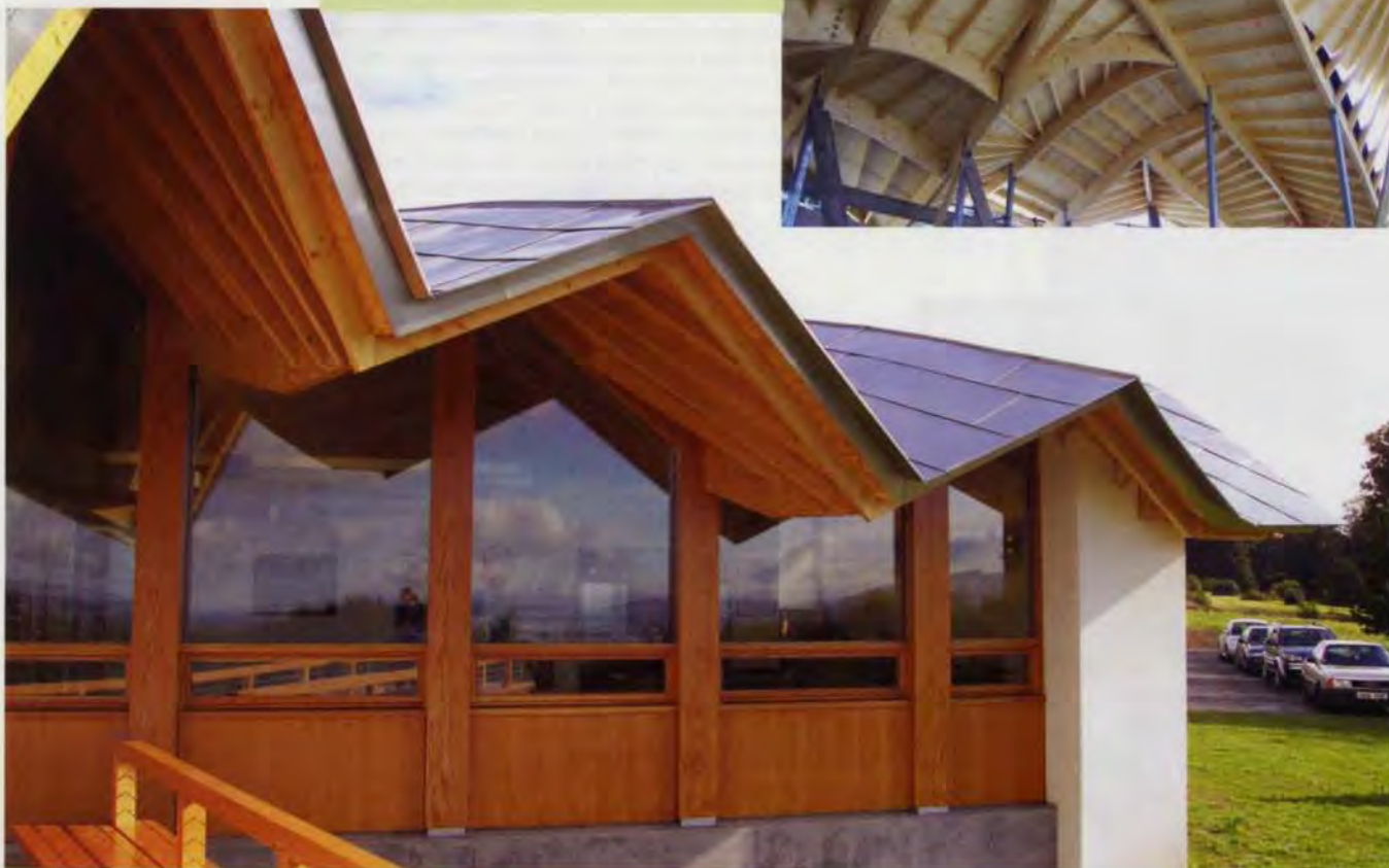
6. The roof has a deep protective overhang.
