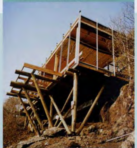
6. Structural frame of a typical unit.
