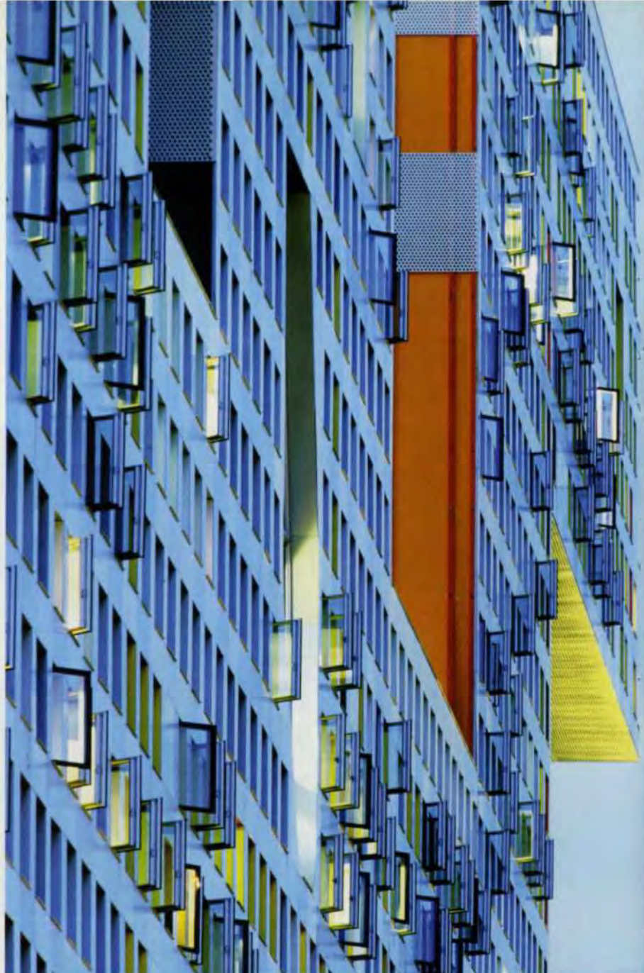
1. Close-up of the south façade, showing the operable windows in use by students in summer.
