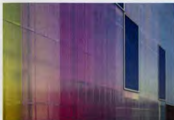
3. The striking bands of colour are now synonymous with the dance studios; the glass selected ensures glare is controlled without reducing daylight.
