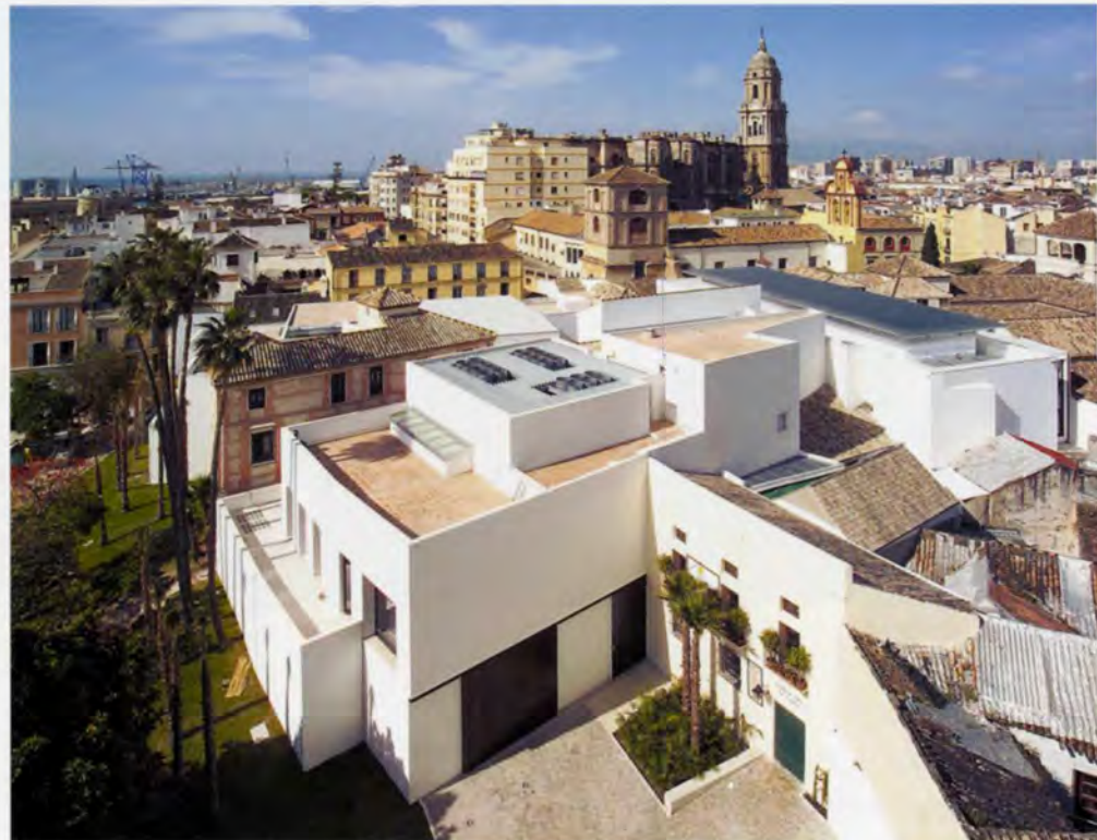
19. The complete museum, with Areas 6 and 7 in the foreground, temporary galleries centre right, and the Palace courtyard on the extreme right.
