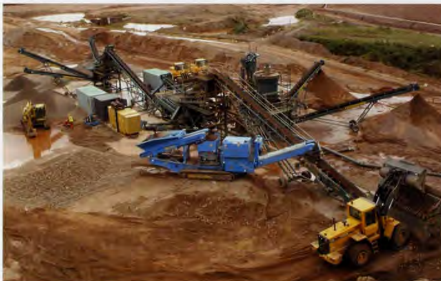
16. Materials processing plant at Weeford Quarry.
