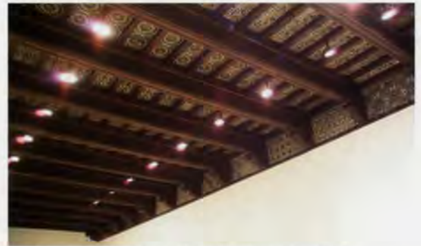
7. Wooden artisan ceiling hung from existing floor slab.
