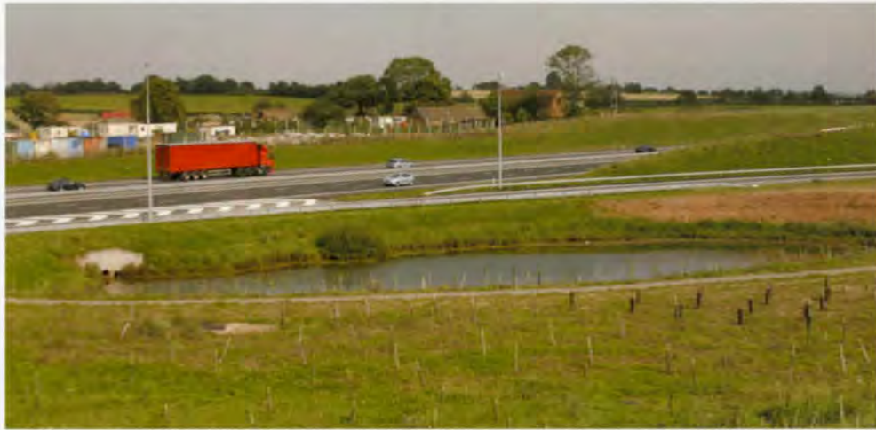
15. Balancing pond near Junction T5.
