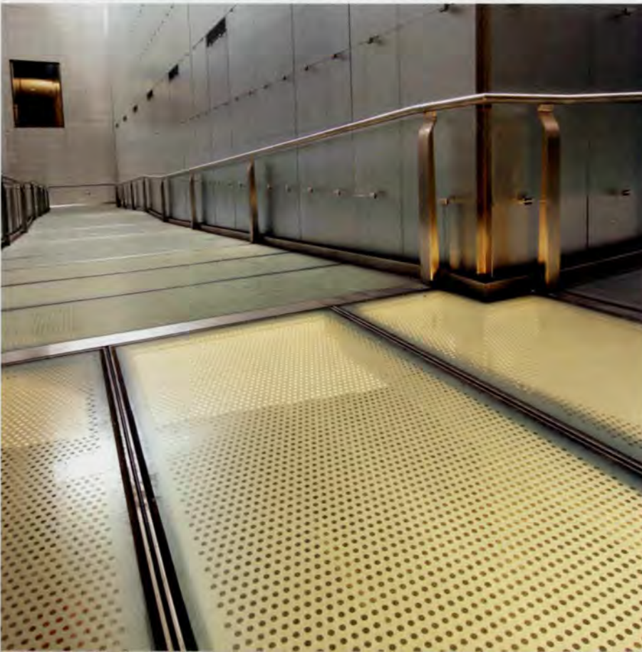
3. The dramatic entry to the new exhibition spaces, showing the steel ramps with glass floor, cantilevered from the side of the exhibition boxes, escalators and circulation spine.
