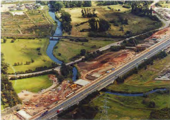
9. Value-engineered structural solutions: extending underbridges for the widening of the M42.
