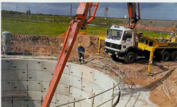
14. Shenstone pumping station.
