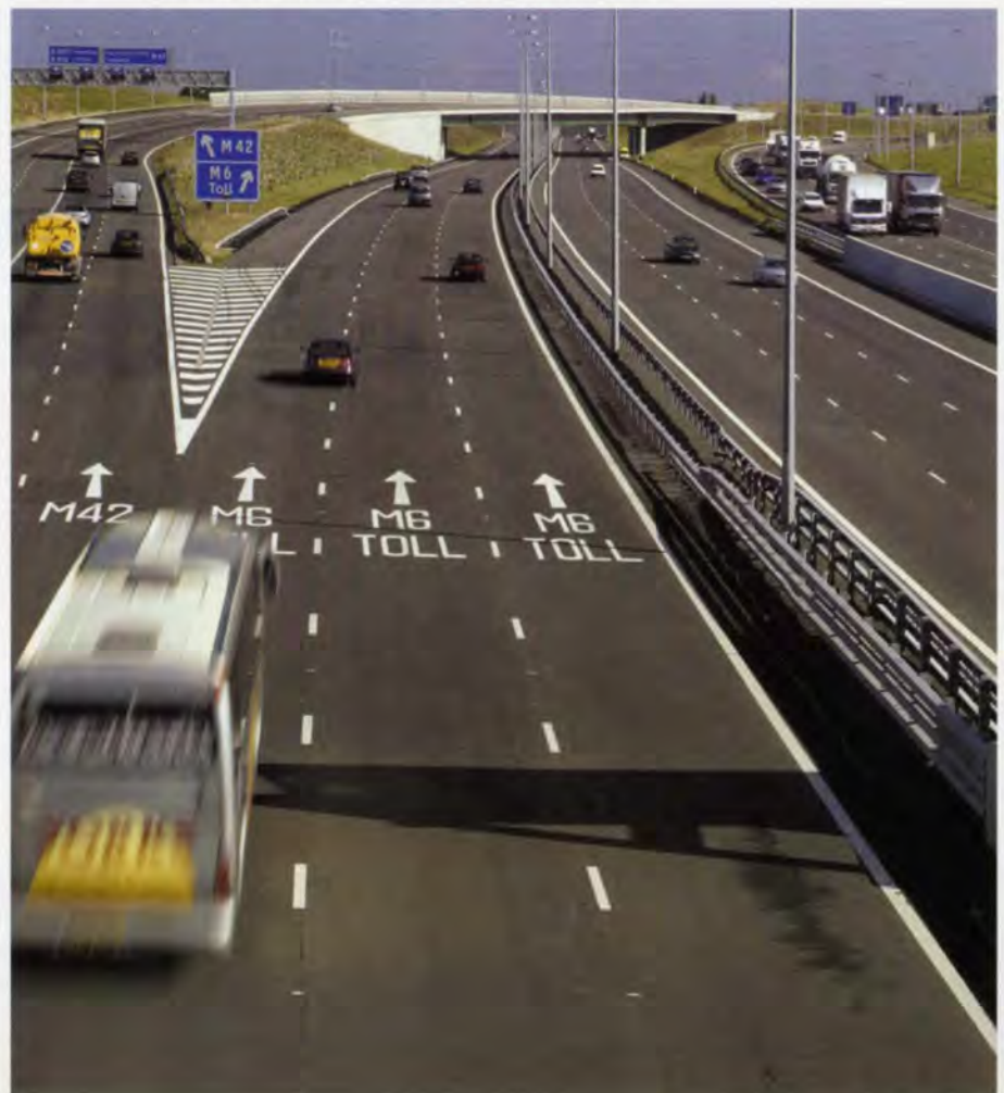
10. M42/M6 Toll junction, where the total width increases to 12 lanes.
