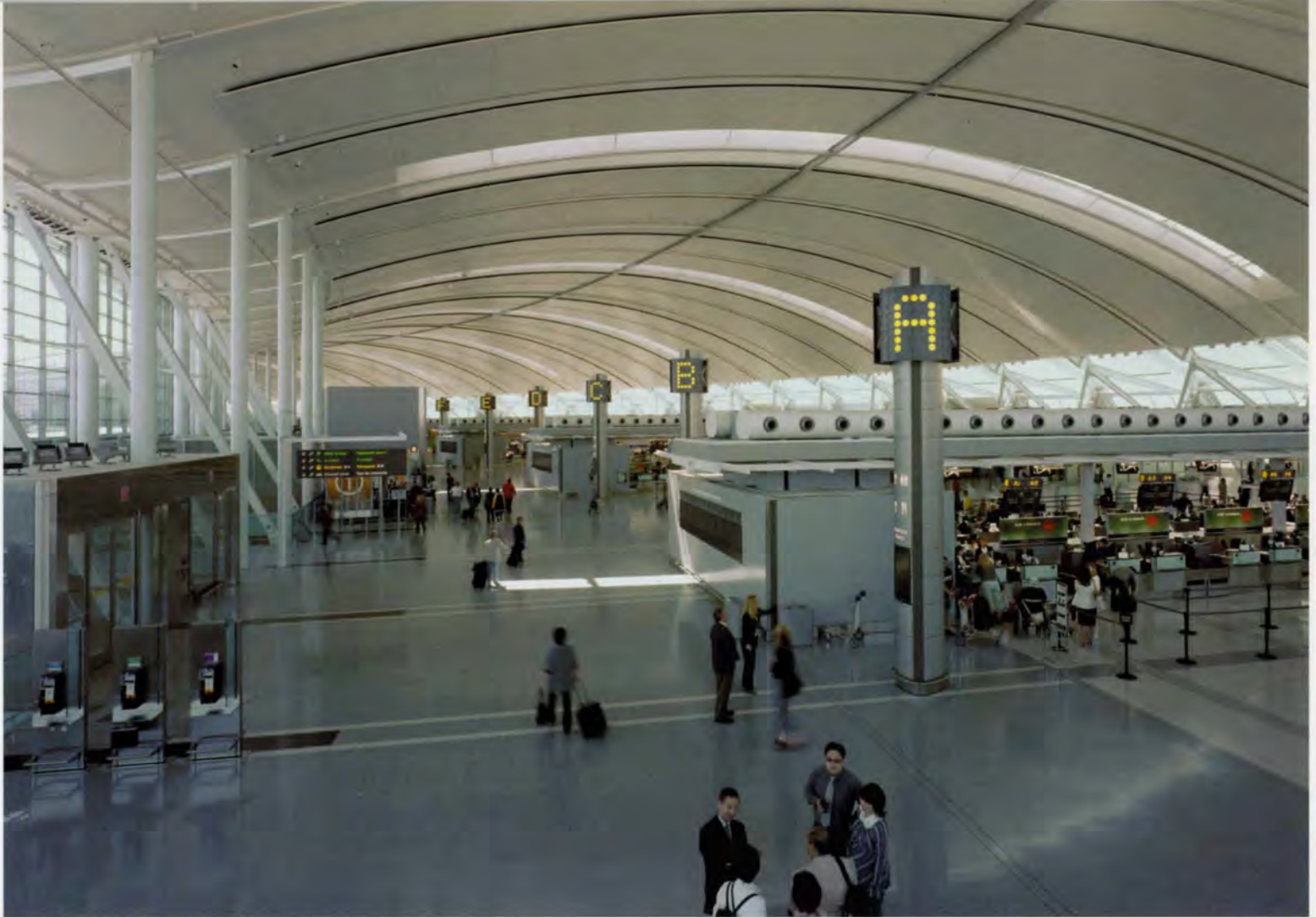
7. The vaulted steel roof soars over the Departures Hall.
