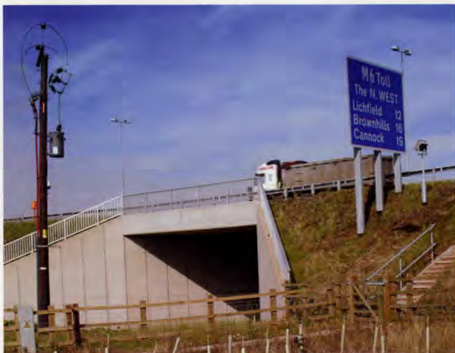
7. Typical concrete underbridge, with new planting in the foreground.
