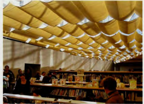
7. Above the Children's Library a fabric shade shields the sun in warm weather and deflects cold downdraughts in cold weather.
