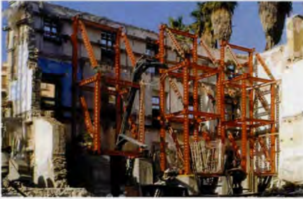
8. Temporary façade support.
