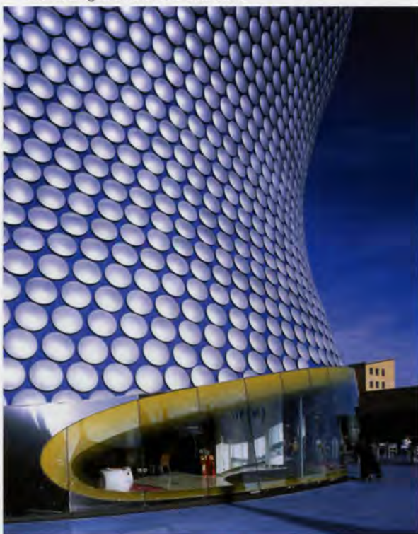
13. Glazing at terrace-level entrance.
