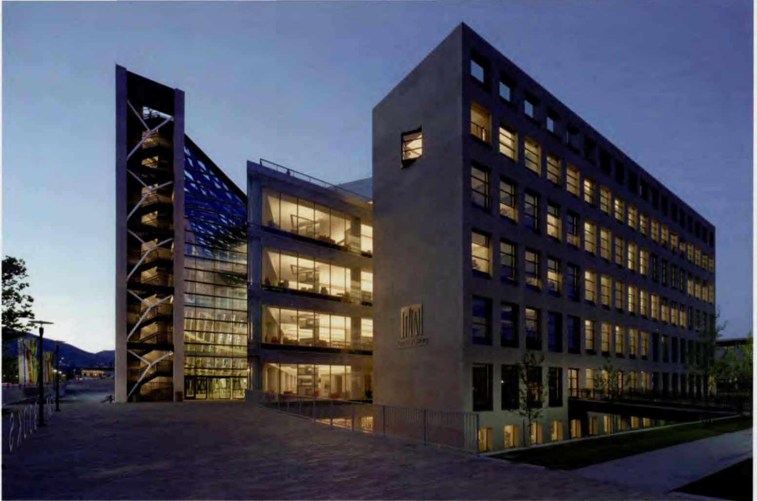
9. The Library is essentially three buildings; from left to right here are the sloping crescent-shaped gallery, triangular stack building and rectangular administrative building.
