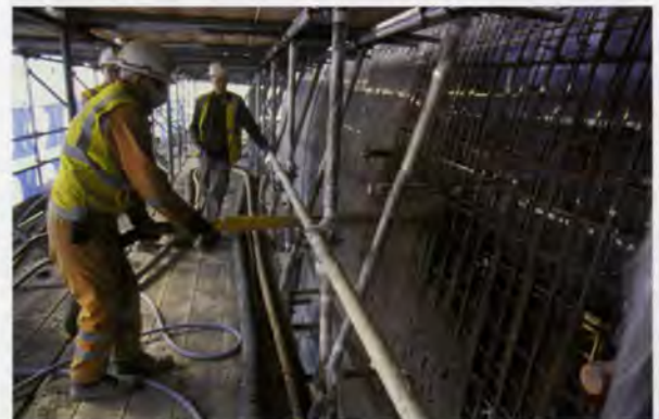
11. Spraying the substrate on site.
