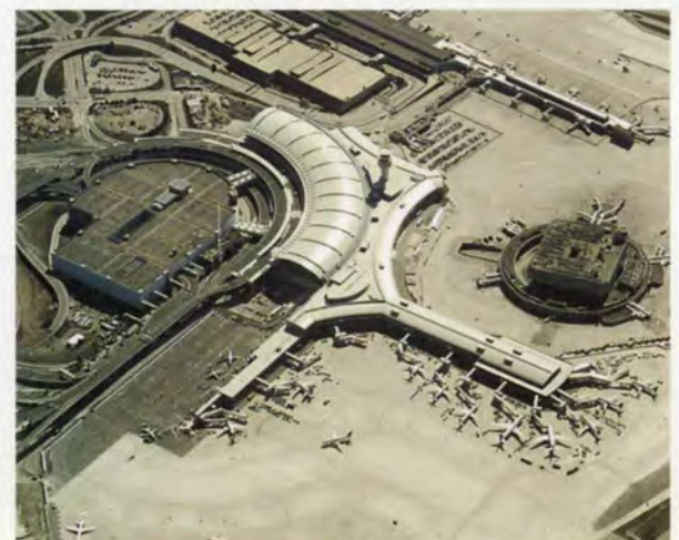
8. Central processor building with Piers D and E mostly completed.
