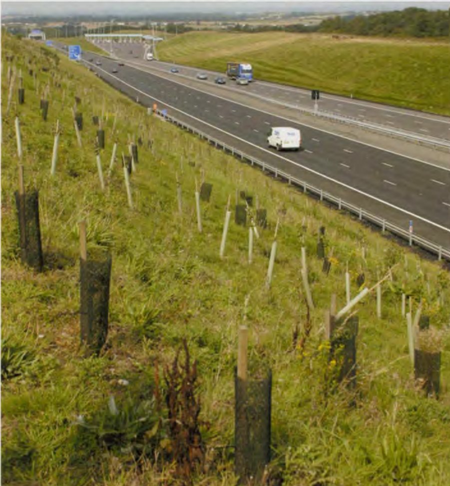
11. New tree planting on the motorway verge near Weeford Park toll plaza.
