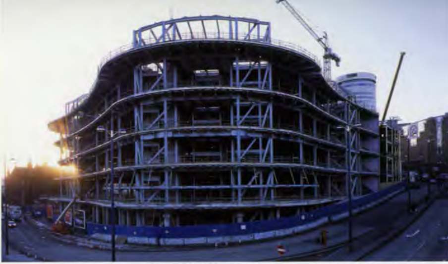
8. External view of completed frame.
