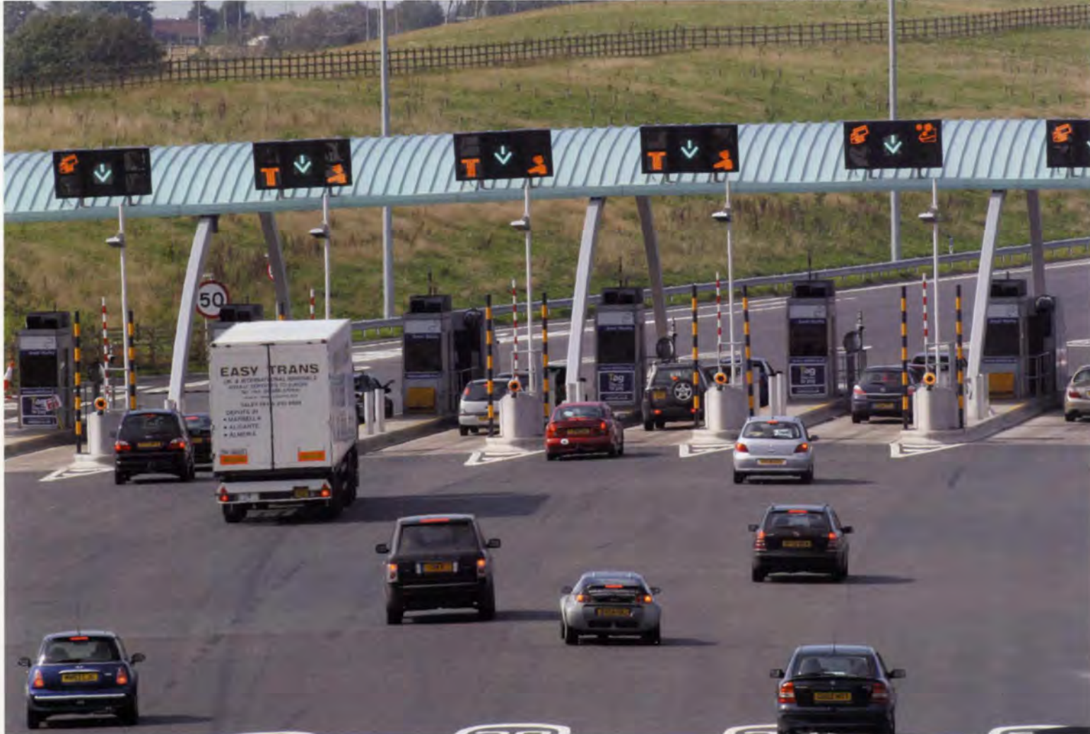
17. Curved roofs and a strong visual identity: toll booths at Weeford Park.
