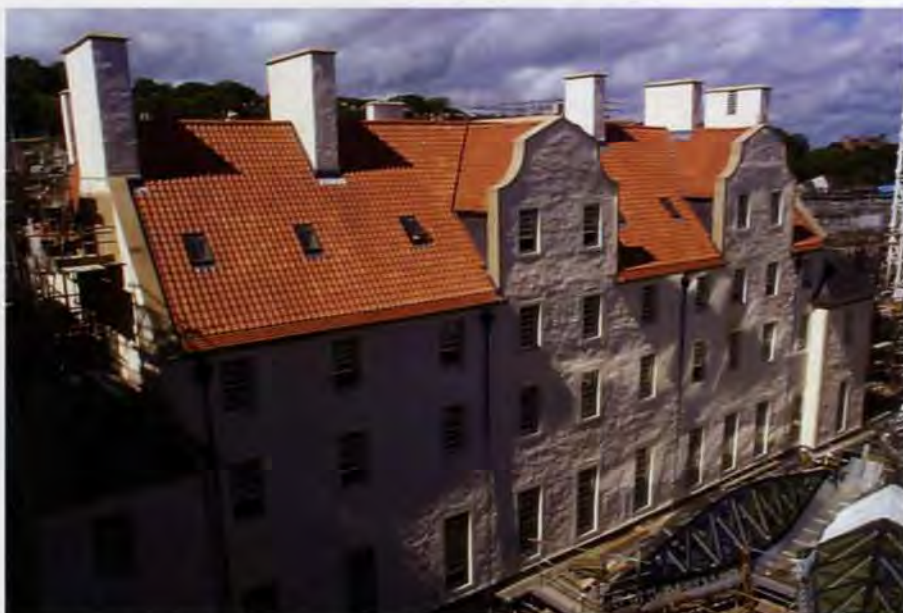
24. Queensberry House after refurbishment.
