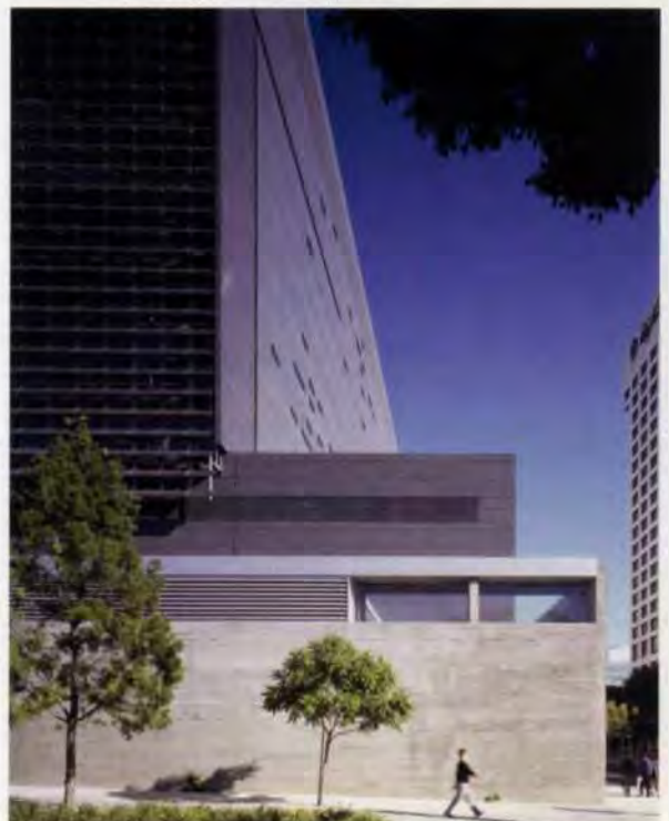
7. View of south-east corner from Second Street, incorporating photovoltaic panels.
