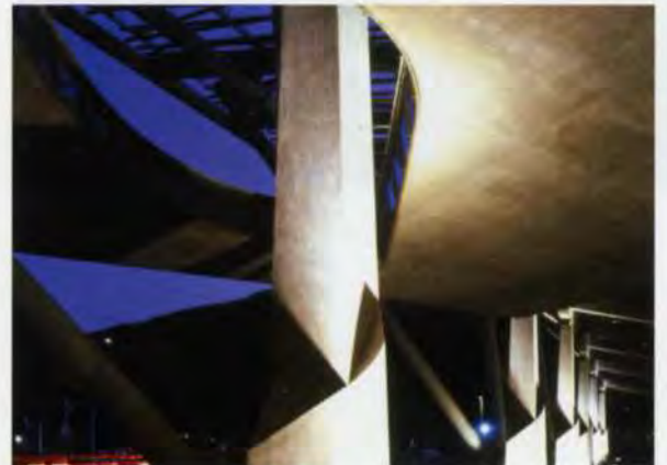
16. 'Flame-shaped' column passing through canopy opening.
