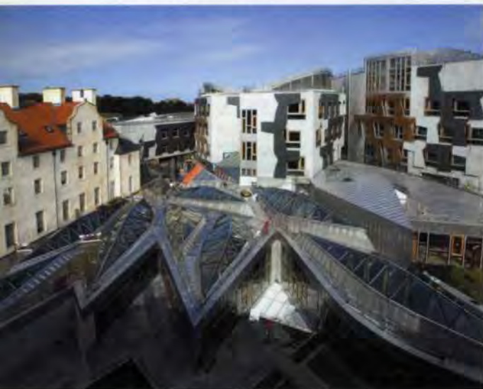
17. External view of foyer roof.
