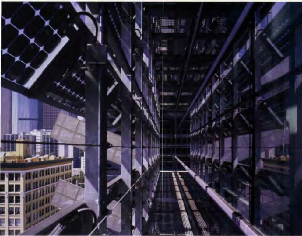
6. View of maintenance walkway on the south façade between glazing and photovoltaic panels.
