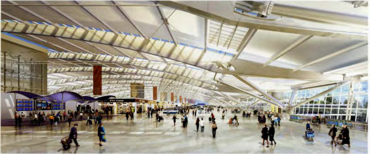
6. Terminal 5 at London Heathrow Airport will use the latest technologies to tailor its wireless infrastructure.
