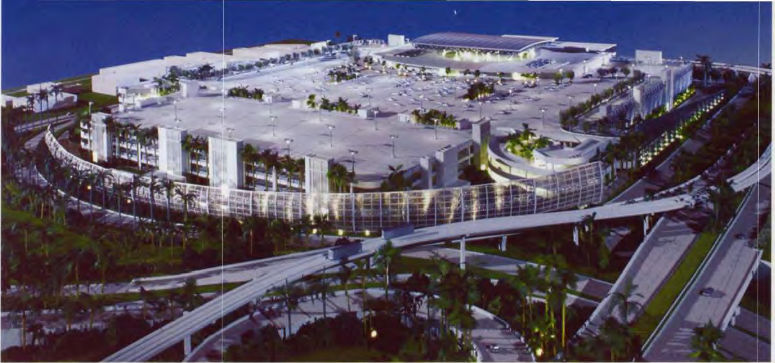
1. The rental car facility from the south-west, with the quick turnaround building in the foreground.
