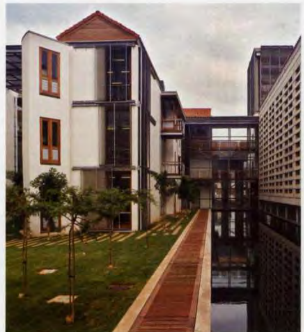
5. Detail of artwork screens on the exhibition gallery elevation, by the top of the Great African Stairs; Constitutional Square and the Court entrance are immediately ahead, and Sections 4 and 5 on the left.
