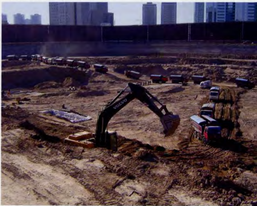
14. Site work begins, September 2004.
