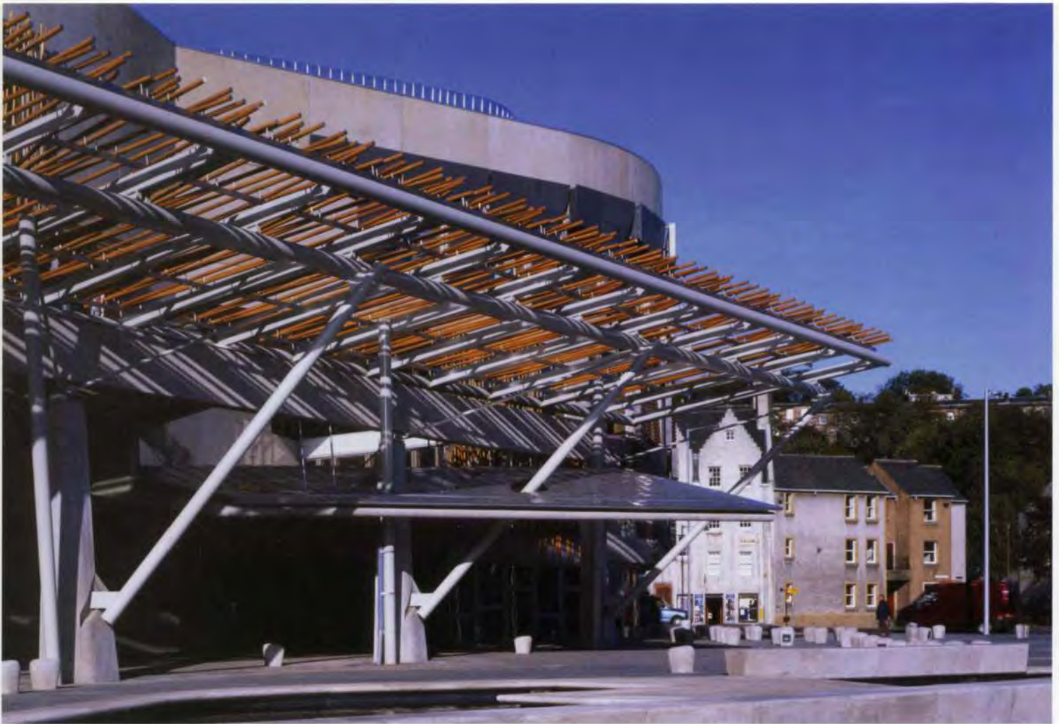
15. Upper and lower pergolas and the north-east canopy.
