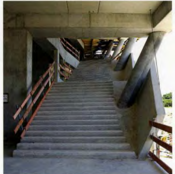
12. Cascading staircase under construction.
