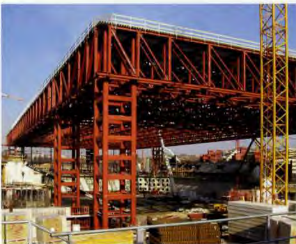
4. "Mega-columns" and roof under construction.
