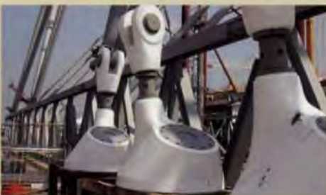
e) Castings on site.
