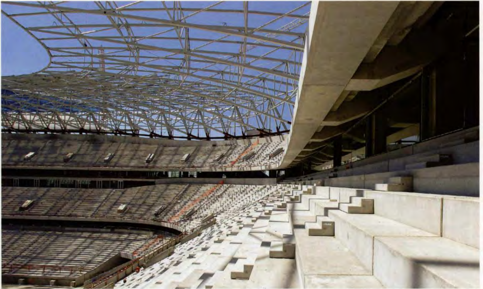
11. Bowl under construction, July 2004.
