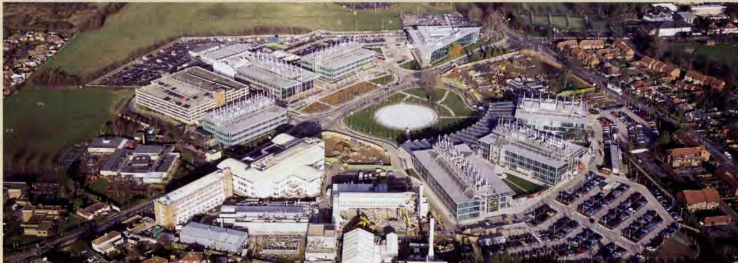
6. By the end of Phase 2, only the buildings in the south-east corner of the site (centre-left foreground) were still served by centralized systems.
