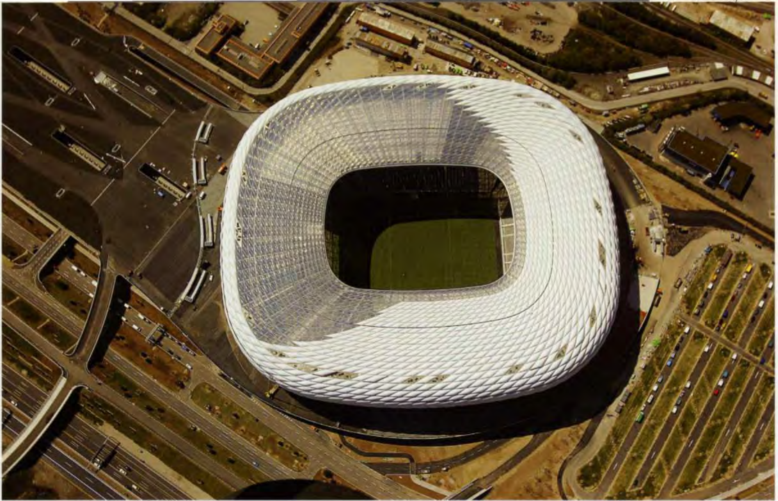
14. The completed stadium.
