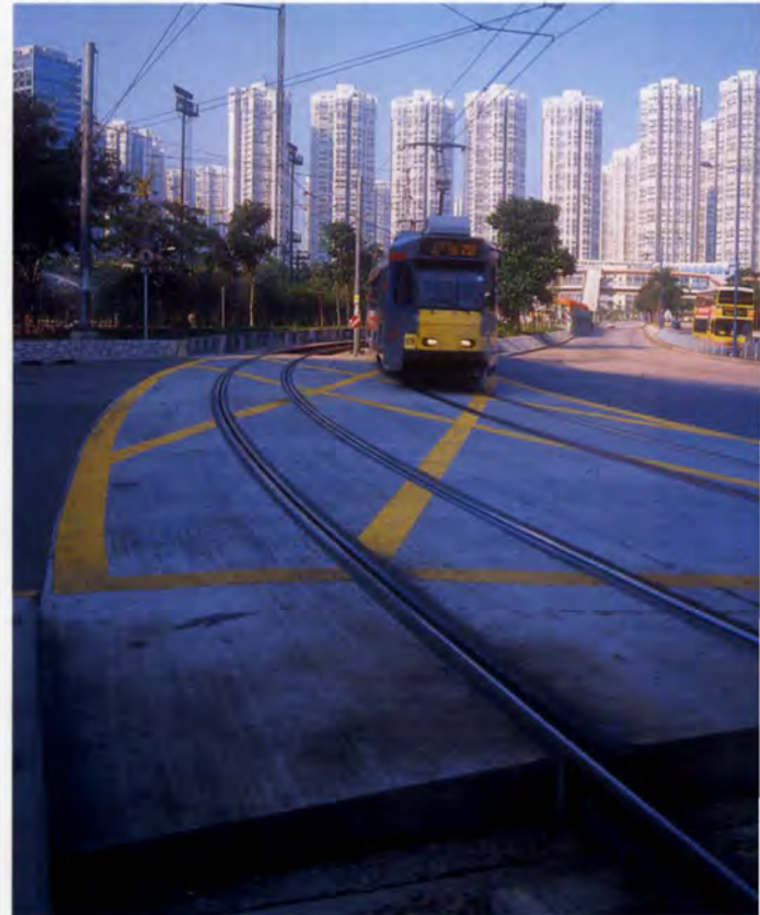
7. Typical road crossing where the trackwork is boxed out within new road slab
