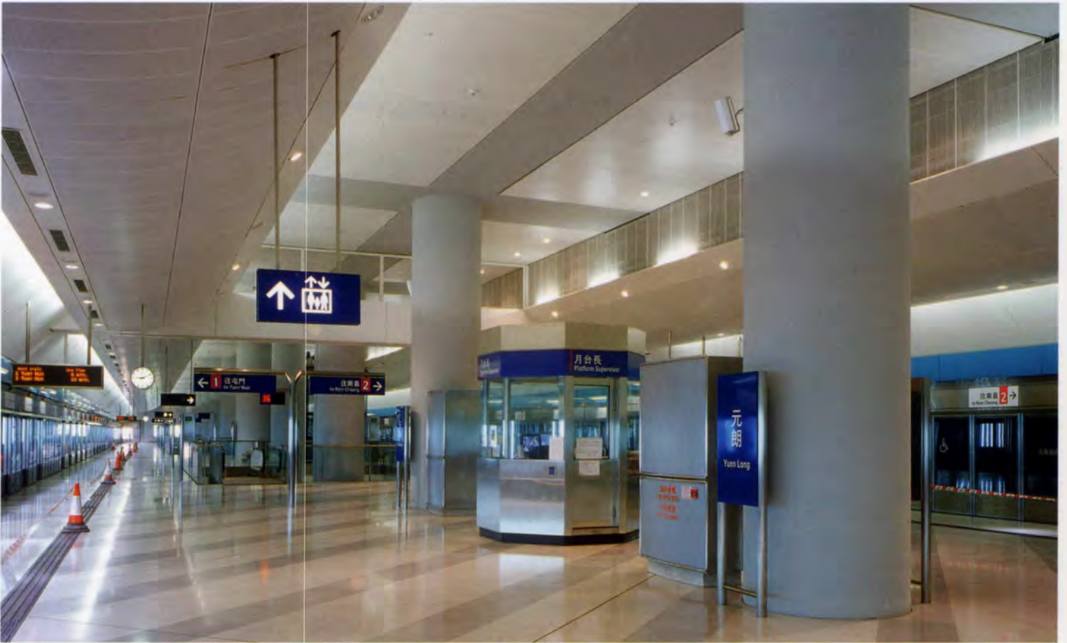
1. Yuen Long Station platform: sound absorption is by absorbent material behind the perforated ceiling panels.
