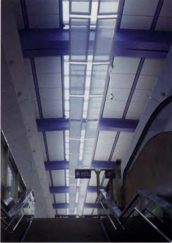
18. Central rooflight at Tin Shui Wai station.
