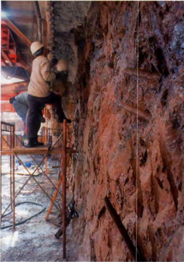
19. Underpinning of diaphragm wall panels.
