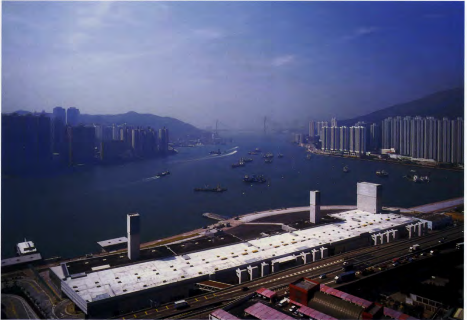
22. North-east elevation of Tsuen Wan West station, with Tsuen Wan bypass in the foreground and Rambler Channel beyond. In the distance is the cable-stayed Ting Kau bridge carrying road traffic into the New Territories to the north, part of the complex of bridges built to handle traffic to and from the new Hong Kong International Airport.
