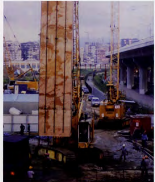
5. De-bonding liner to barrette test.
