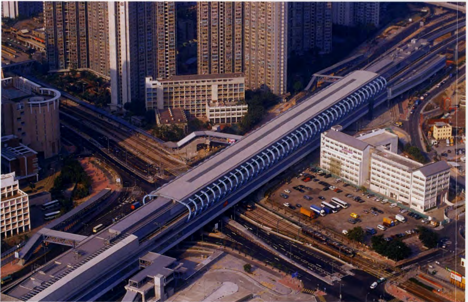
21. Roof cladding at Tin Shui Wai station.
