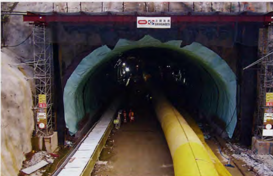
1. The Tai Lam tunnel north portal.
