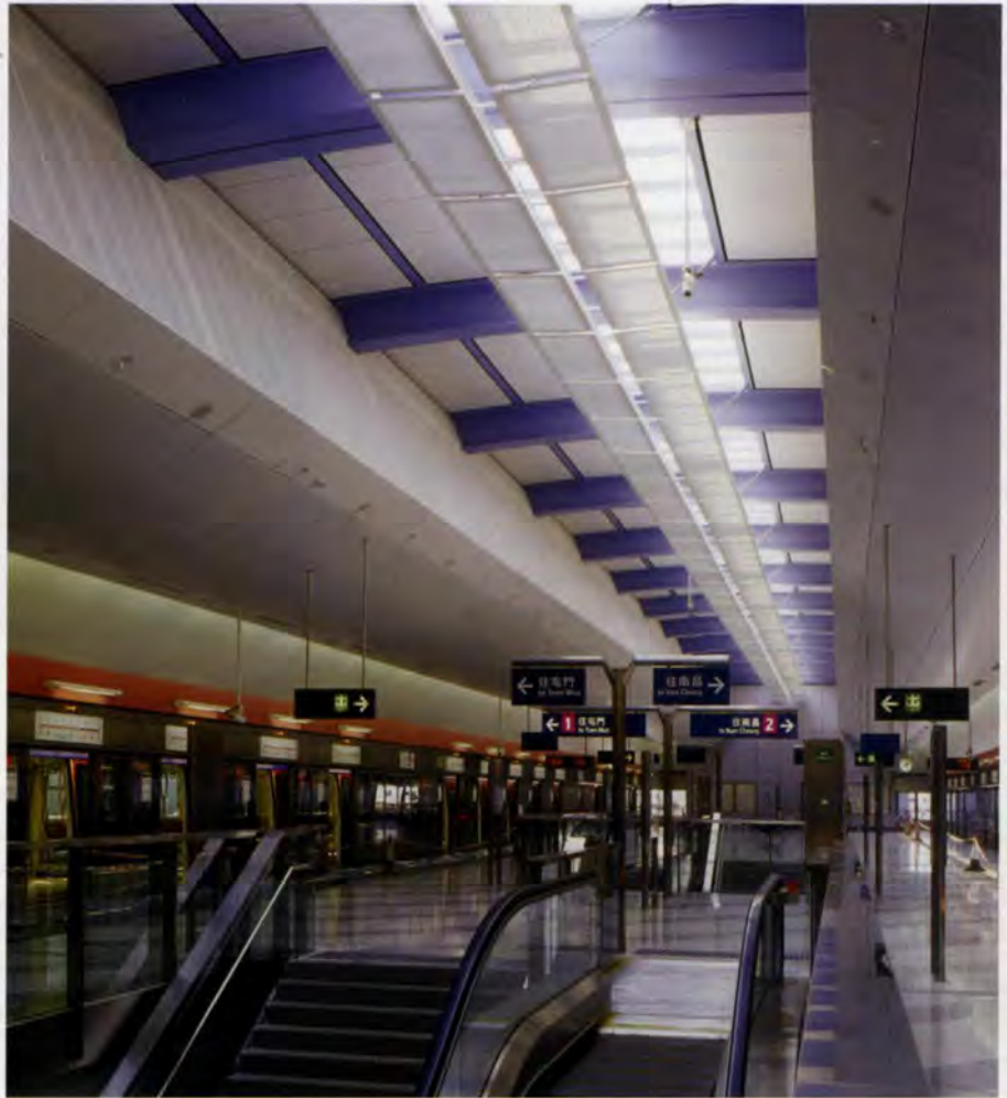
5. Acoustic ceiling panel at Long Ping station.
