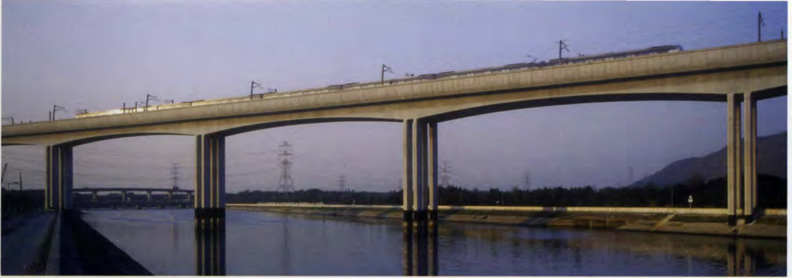
1. Long viaduct spans across the Kam Tin River.
