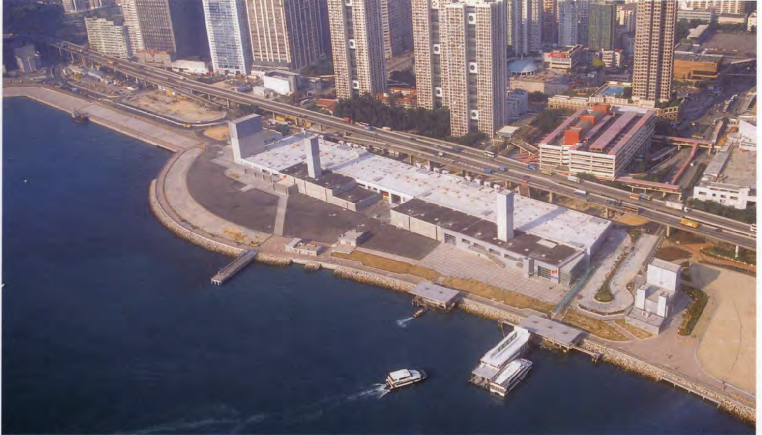
1. South-west elevation of Tsuen Wan West station from the air.
