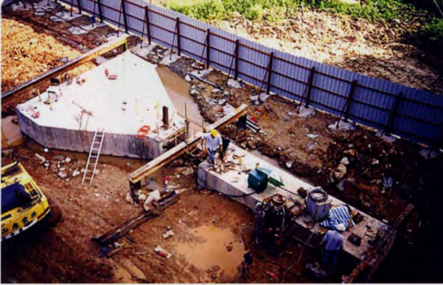
3. Lateral load test on pile groups.
