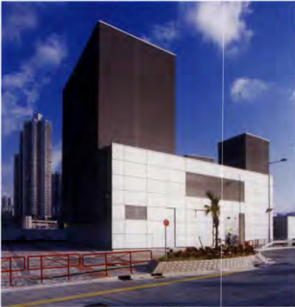
15. Southern transformer building.
