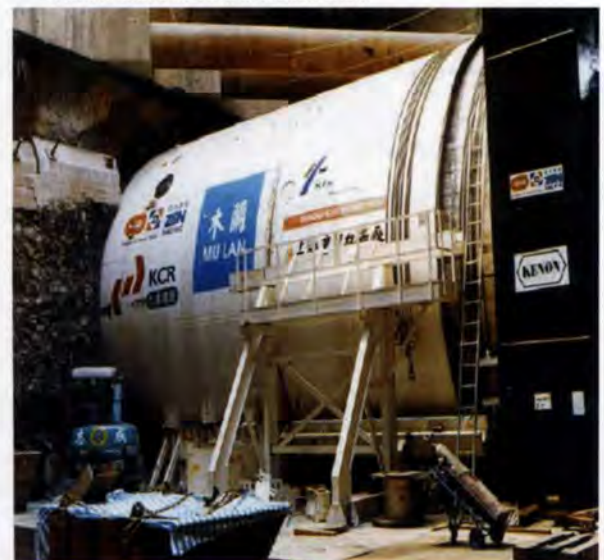
3. Front shield of TBM in launch shaft.
