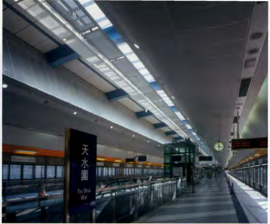
3. Acoustic ceiling panels at Tin Shui Wai station.
