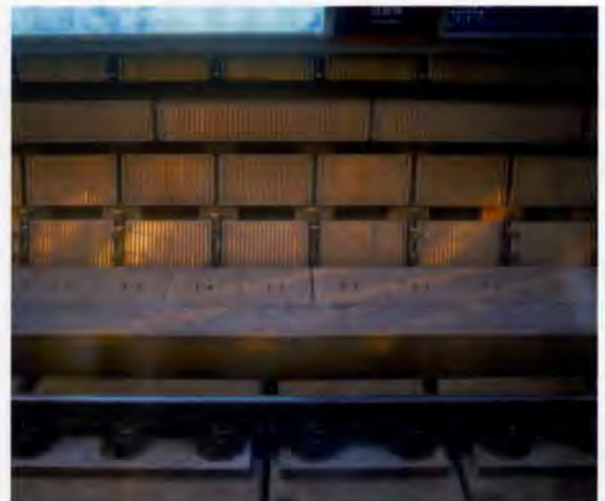
8. Acoustic panels on the parapet.
