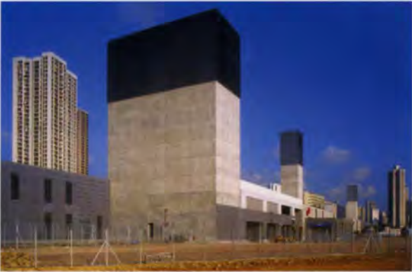
10. View from the north-west; façade to be enclosed by future property development.
