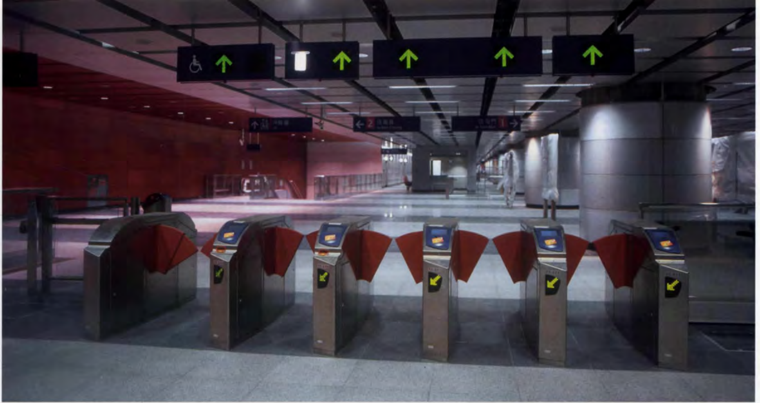
5. The concourse level, showing columns designed to carry future property development above the station.
