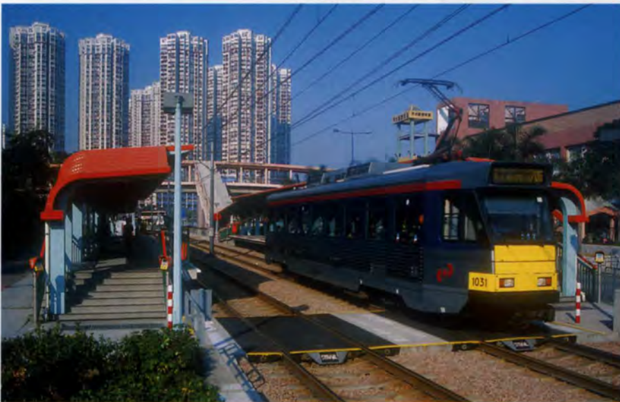
2. Typical light rail stops match those on the existing system - also designed by Arup, in the mid-1980s. This stop is at Tin Wu.
