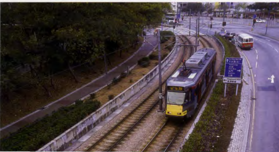
5. This view between the stops at Tin Wu and Ginza shows the 8m wide reserve in which the LRT extension was built.
