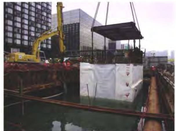
21. Installation of precast seawater pump chamber by barge-mounted crane.
