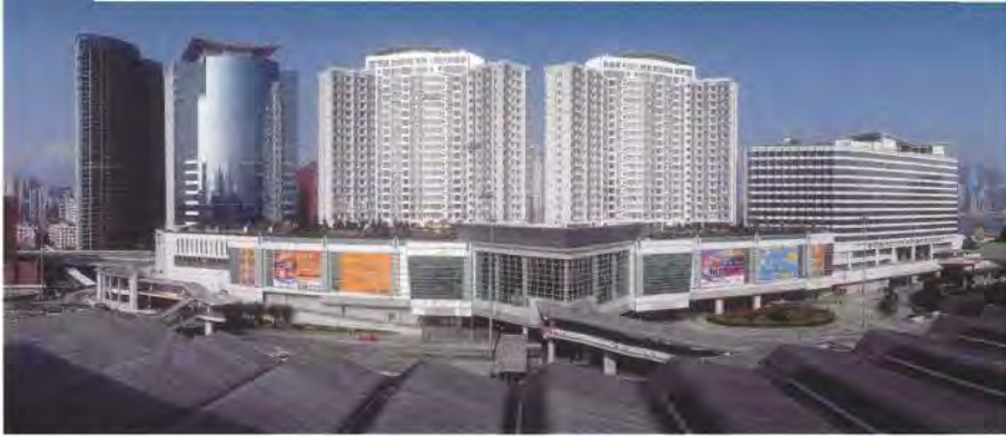
6. The Metropolis development alongside Hung Hom station.
