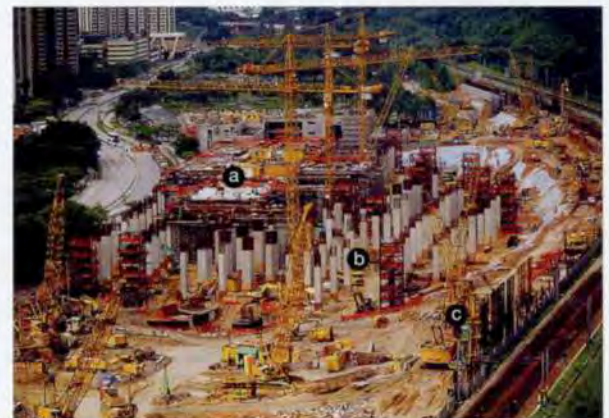
11. (a) Podium slab (b) podium columns, (c) East Rail protection.
