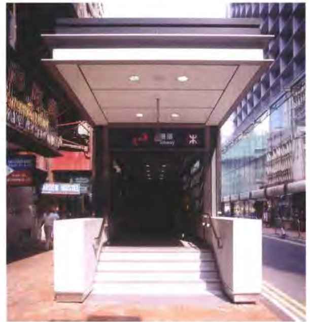
17. Entrance to subway in Mody Road.
