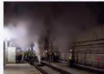
12. Initial release of cold smoke for twin-track tunnel test.
