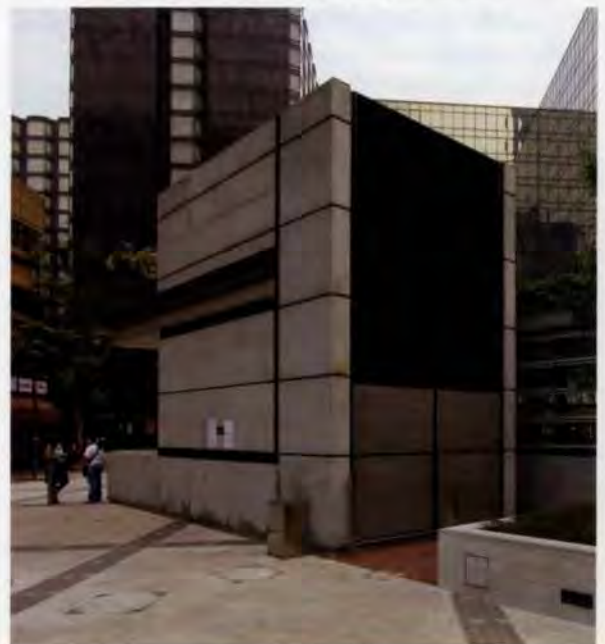
3. Exhaust-air vent shaft integrated with passenger lift.
