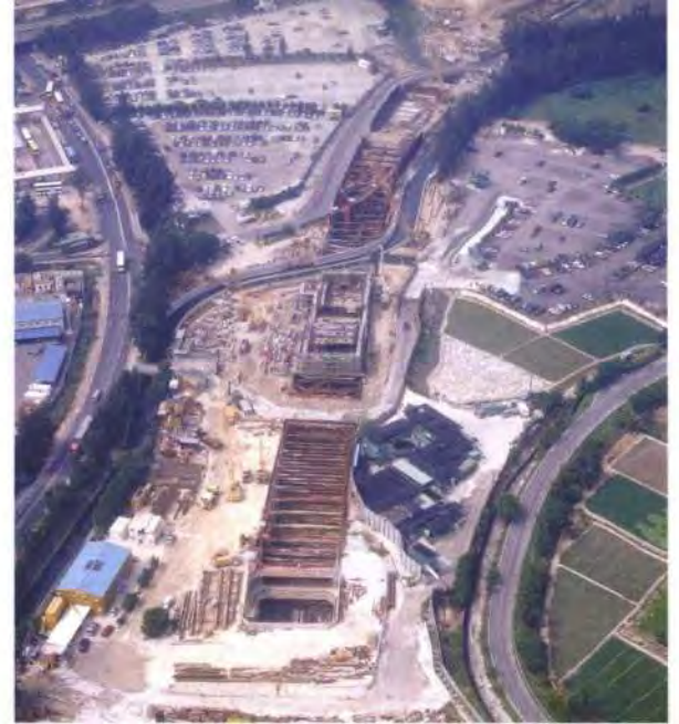
16. Aerial photograph of west approach under construction.
