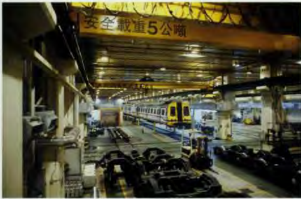
3. Ho Tung Lau maintenance centre.
