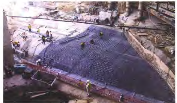
12. Reinforcement fixed for ballast trough base slab.
