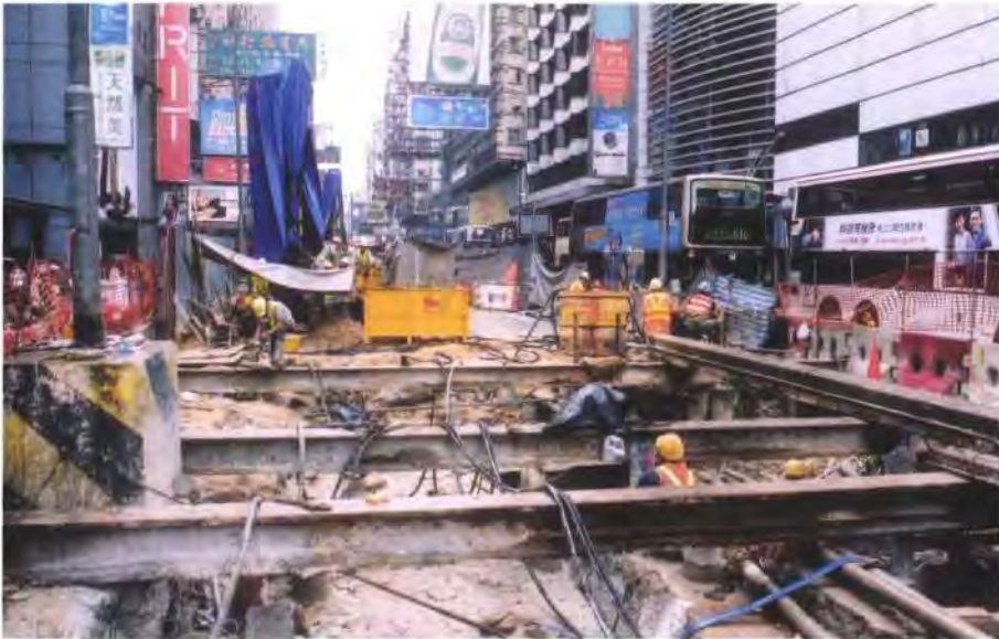
16. Initial excavation and decking supports for Nathan Road crossing.
