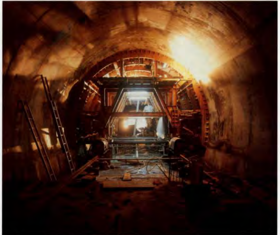
15. Lining to completed Signal Hill tunnel.
