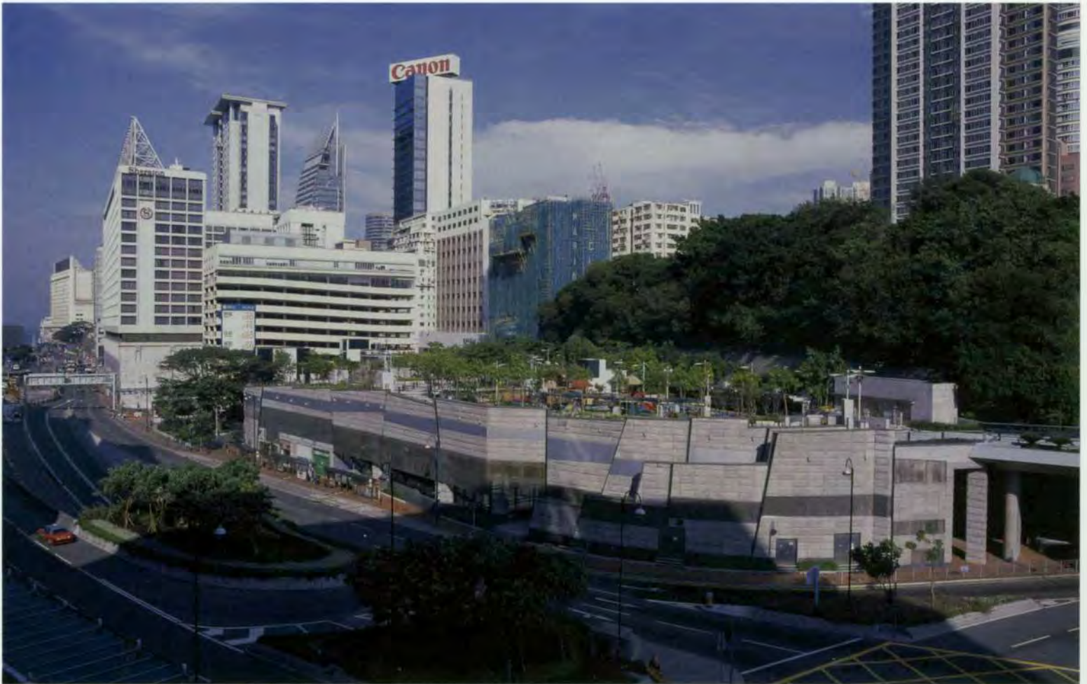
22. Station at foot of Signal Hill, with re-provisioned Middle Road children's playground at elevated deck level.
