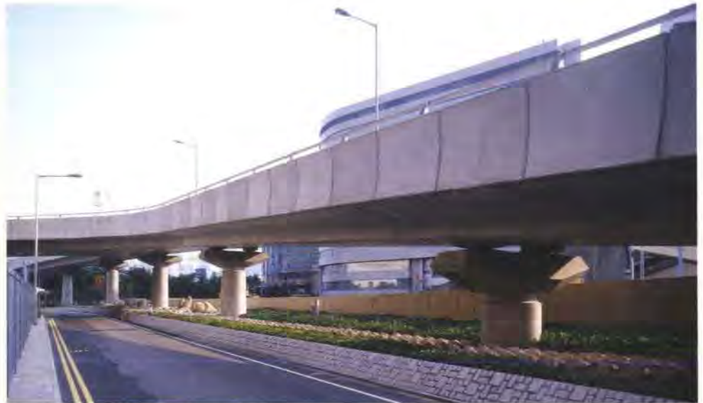
4. New elevated access road to IMC and freightyard.
