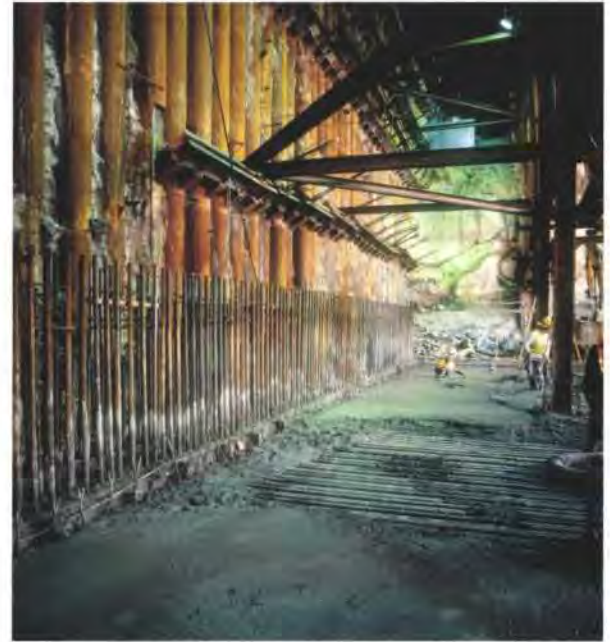
12. Temporary strutted and anchored perimeter retaining wall construction.
