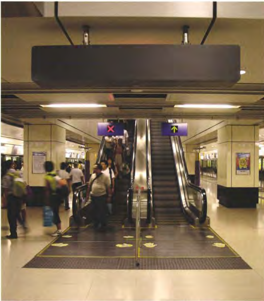
20. The station island platform, showing twin column arrangement flanking escalators.
