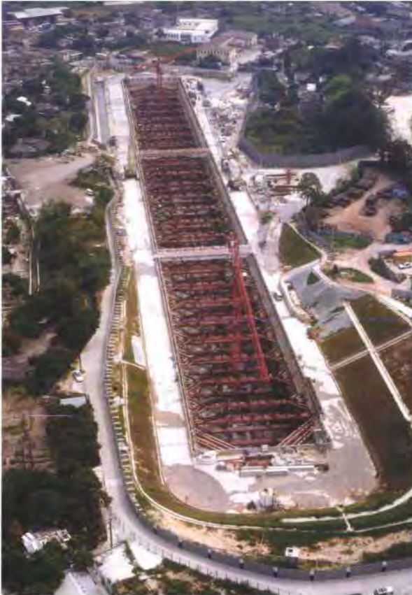
13. Aerial view of Kwu Tung during construction.
