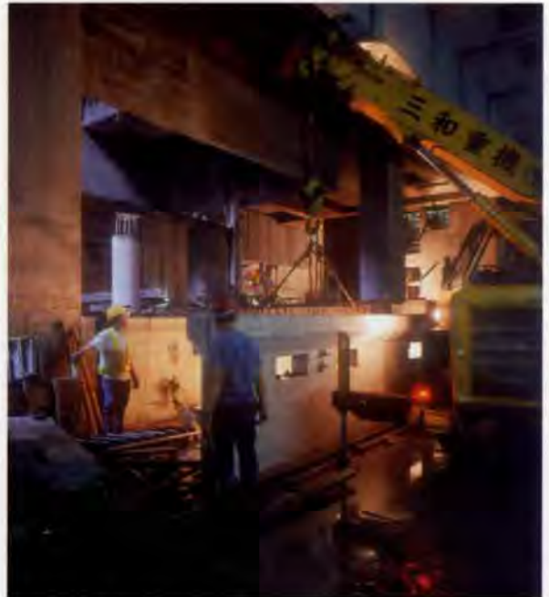
16. Installing a precast platform wall unit.
