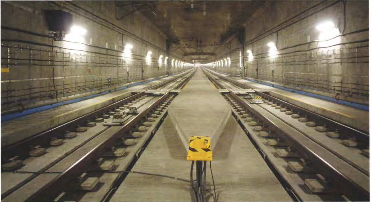
14. The completed twin-track, single-compartment tunnel.
