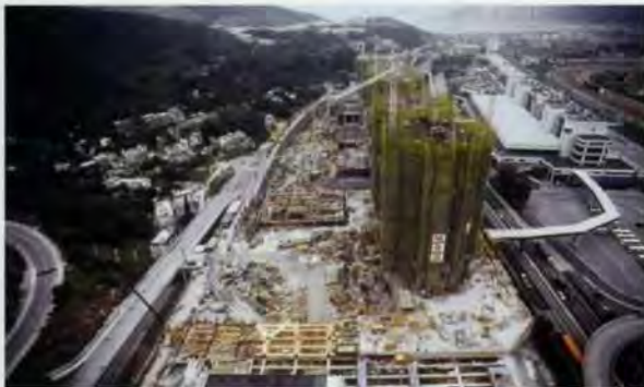
4. Development under construction above Ho Tung Lau maintenance centre.
