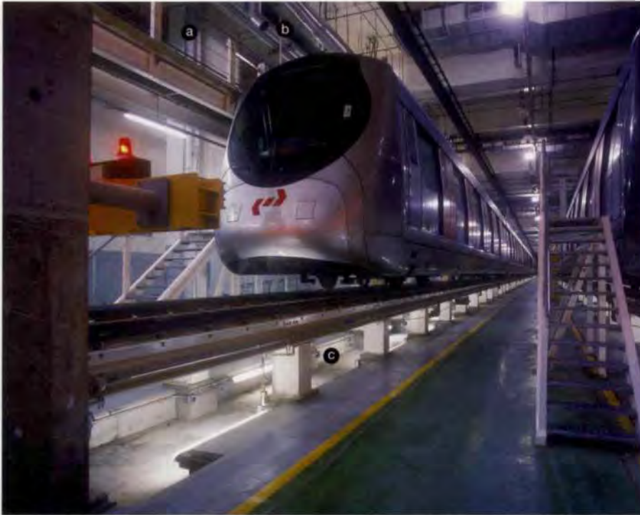
3. Running maintenance track - (a) high level access, (b) spot cooling ducts, (c) maintenance pit.
