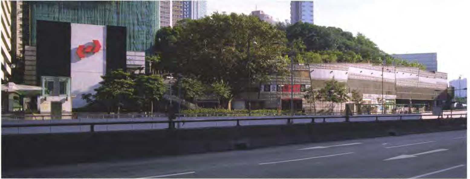
1. The station from Salisbury Road.
