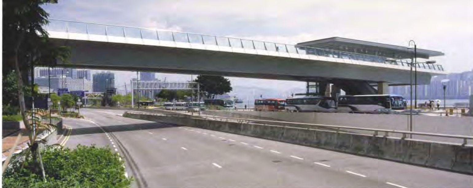
2. Salisbury Road access bridge.
