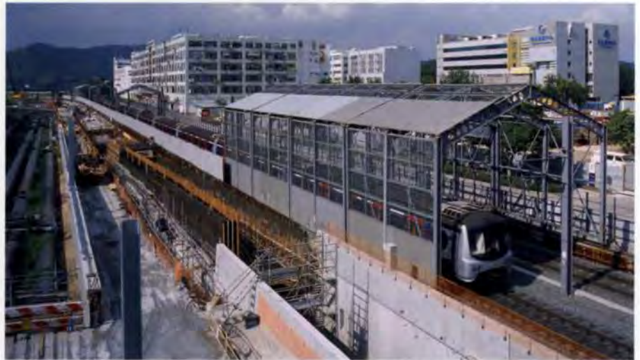
4. East approach during construction, showing temporary protection frames.
