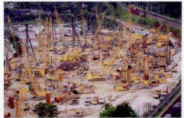
10. Piling plant at peak production.
