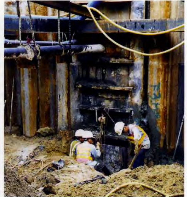
10. Lagging installed ahead of main excavation to reduce risk of flooding.
