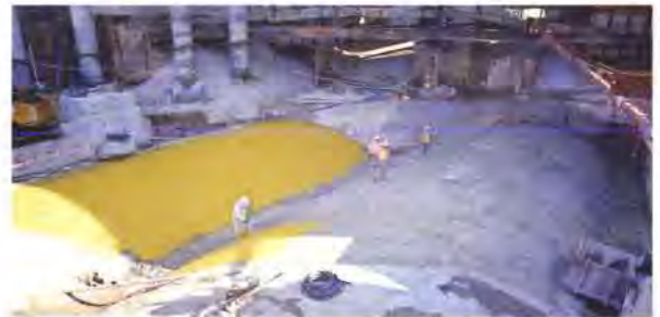
11. Additional waterproof membrane applied to CHT roof.
