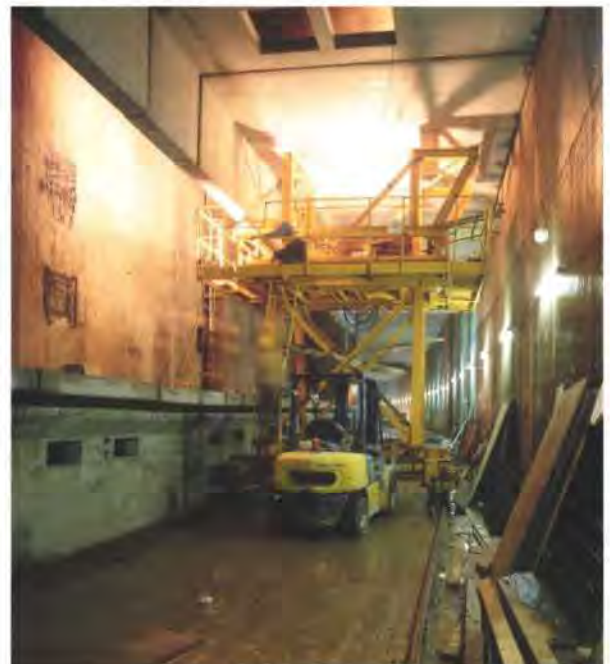
14. Positioning overtrack exhaust duct units.
