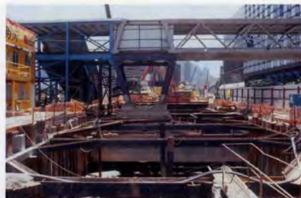
5. Underpinning of footbridge with transfer beams.
