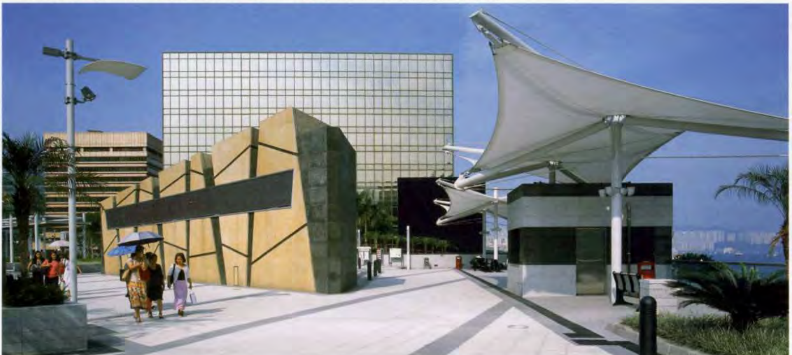
1. Wing On Plaza garden deck. On the left is the vent structure serving the public transport interchange below.
