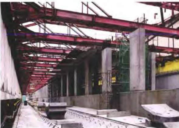
14. Kwu Tung under construction.
