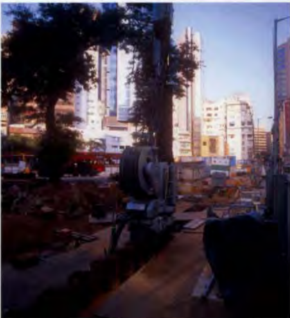
12. Giken SC100 Super Crush Piler in Mody Road.
