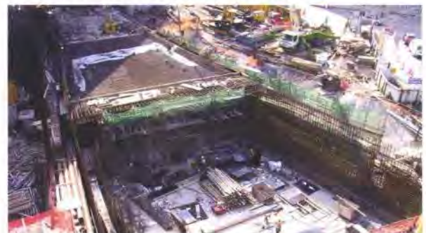
13. Tunnel walls and roof cast monolithically.
