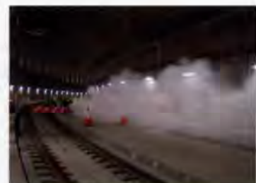
13. Tunnel ventilation system pushing smoke towards Hung Hom ventilation building.
