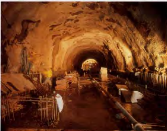
14. Signal Hill tunnel excavation.
