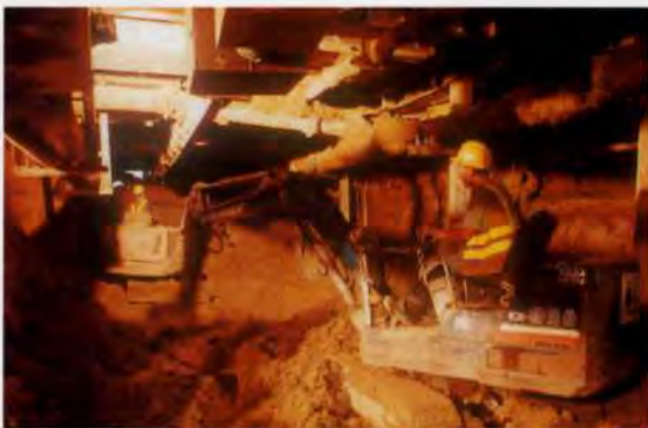
13. Excavation beneath the road deck.
