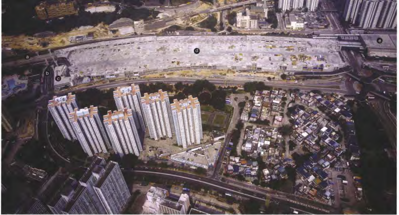
13. (a) East Rail lines, (b) podium access ramp, (c) administration building and training centre, (d) podium with completed maintenance centre below, (e) Tai Wai station.
