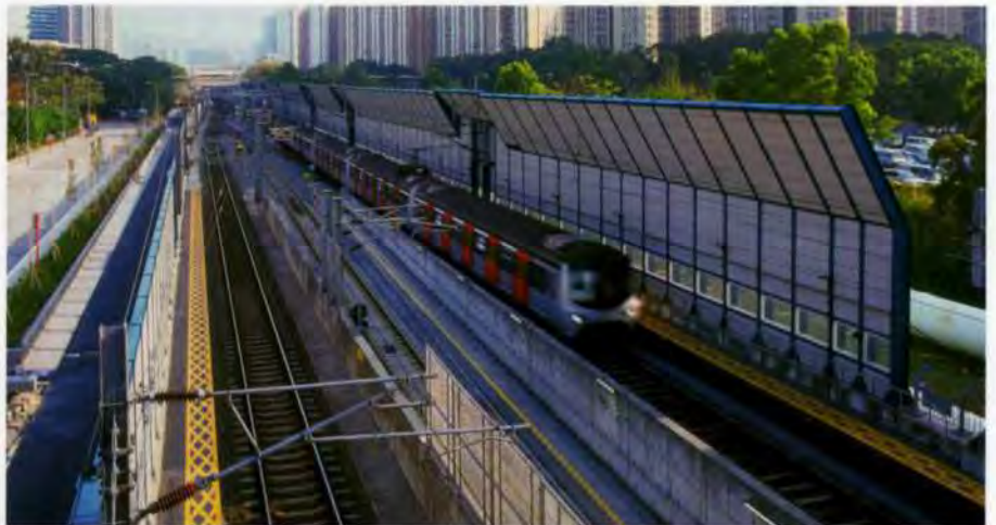
5. East approach with noise barriers in position.
