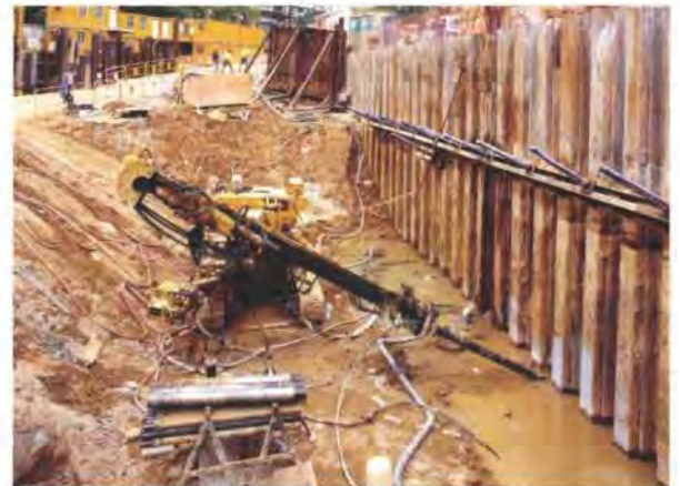
13. Stressed anchor system at Wing On Plaza garden excavation.
