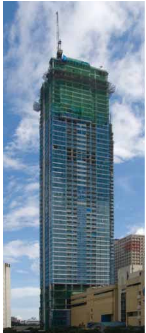
19. The St Francis Shangri-La Place development under construction, October 2008.
