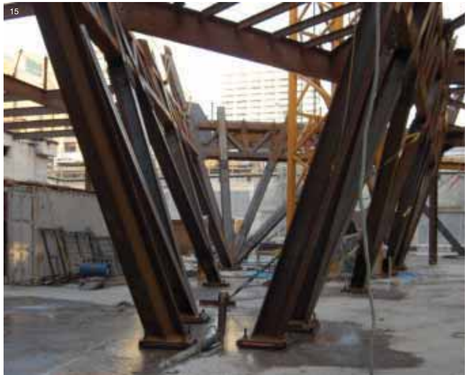
12. New frame adjacent to original building. 13. Crystal 5 spanning the original building. 14. Frame tailored to suit cladding arrangements. 15. Frame springing from "blockbuster" basement level.
