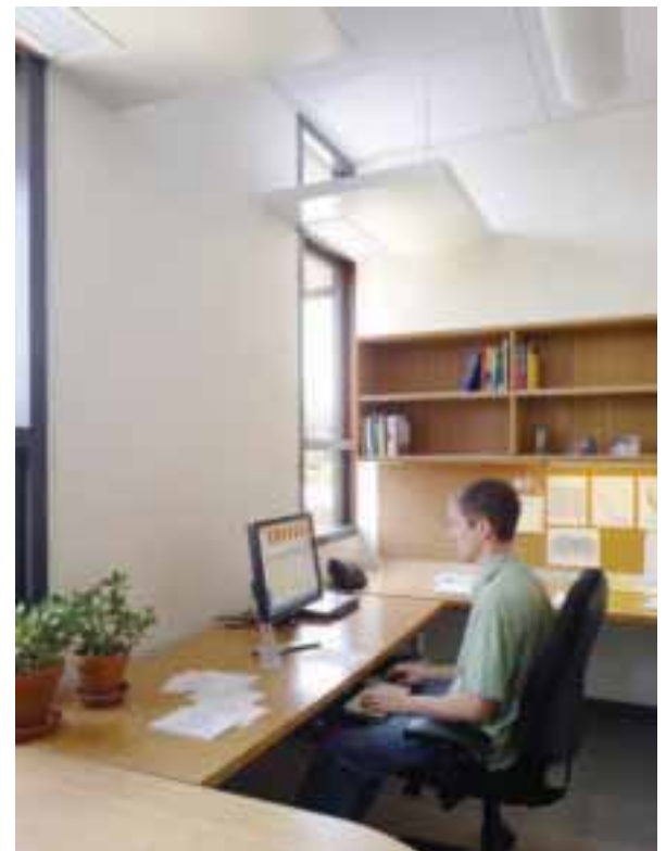
18. Engineered light shelves and exterior shades optimise the provision of daylight in the building,
