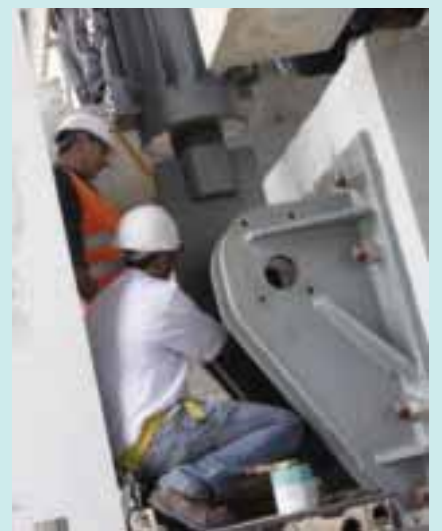
17. Contractor fits first damper to lower anchor frame.
