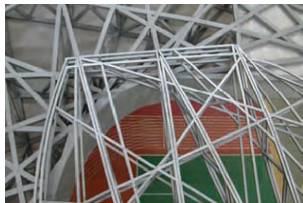
4. Continuity between fixed and retractable roof.
