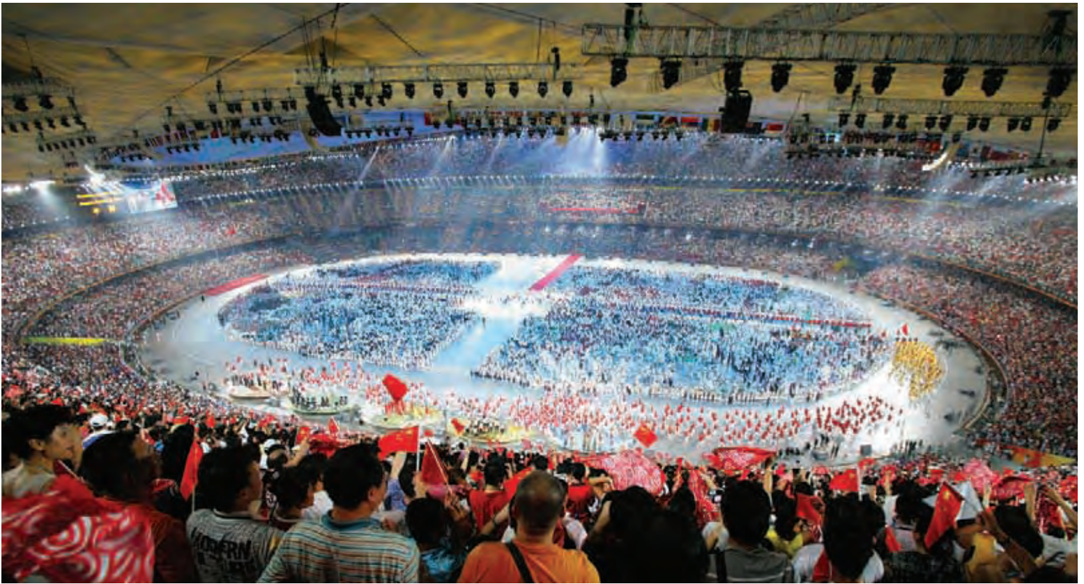
9. The continuously-curved form of the seating tiers provides better viewing standards for all spectators .
