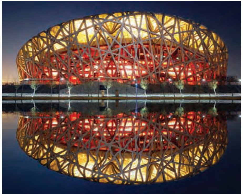
14. The structure, painting, and lighting create an impressive effect, especially at night.
