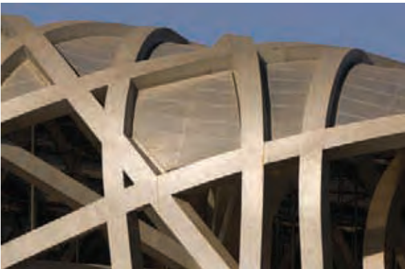
2. Outer ETFE cladding.
