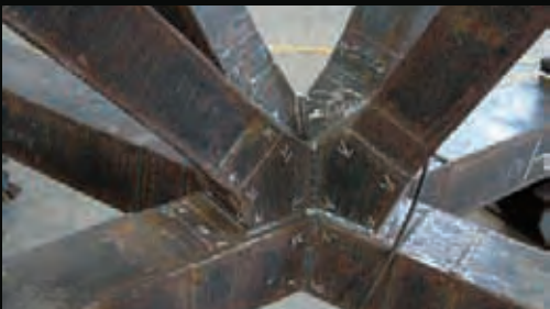
12. Double K-node of a primary truss.
