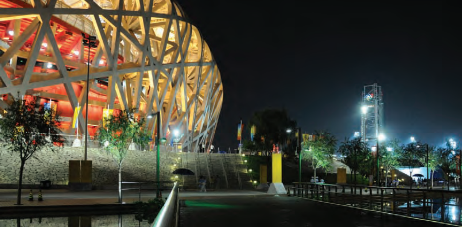
1. Exterior lighting is kept to low levels to enhance the lantern concept.
