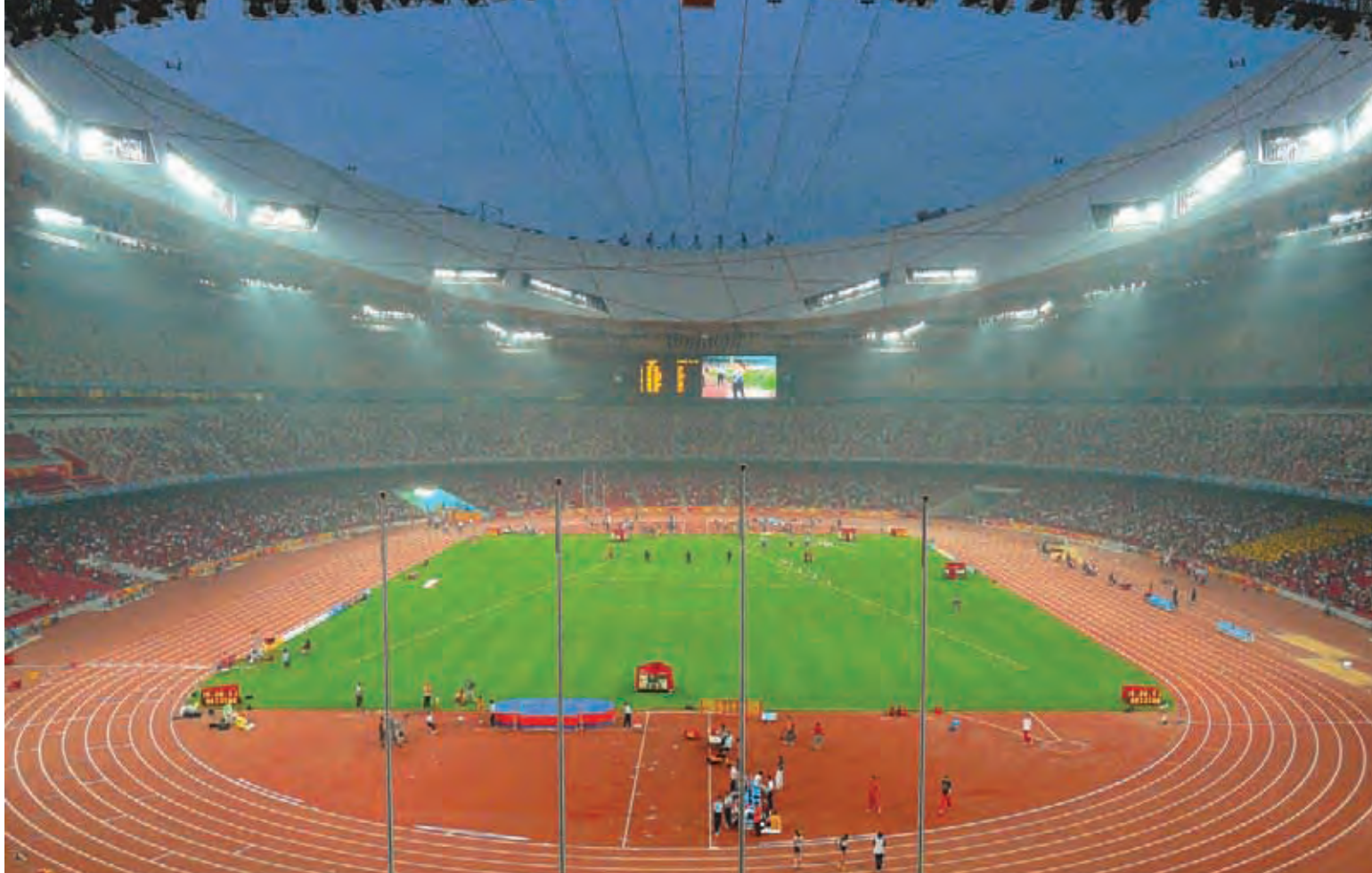
1. The final design allowed a larger opening above the pitch and a reduction in the amount of steel used in the fixed roof.
