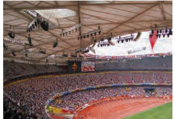
10. The acoustic reflectivity of its envelope and lining below the roof membranes, all give the Stadium an outstanding acoustic quality.
