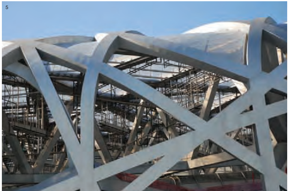
1. Erection of a roof member. 2. Construction of tribune beam of upper tier. 3. Installation of outer column base. 4. Roof main trusses installed for the ring truss portion. 5. Close-up of the eave portion of the roof/façade, showing the curved and twisted structural members.
