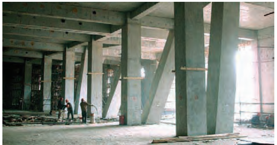
7. Inclined columns in concourse area.
