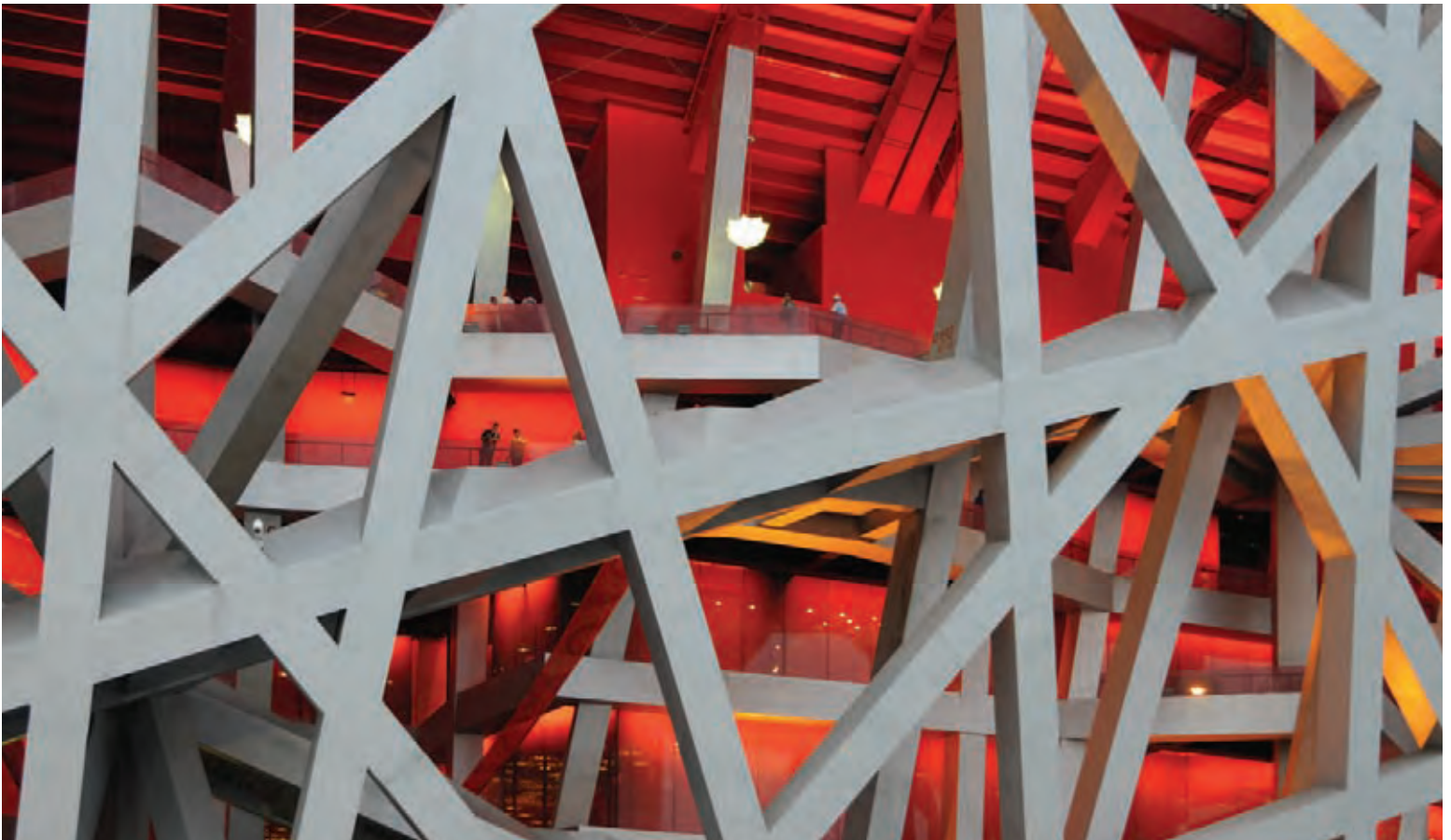
4. “Wall washing” of the bowl surface and glass walls, the pendant lighting and the accent spotlights, all combine to create the ambience of the concourse levels.
