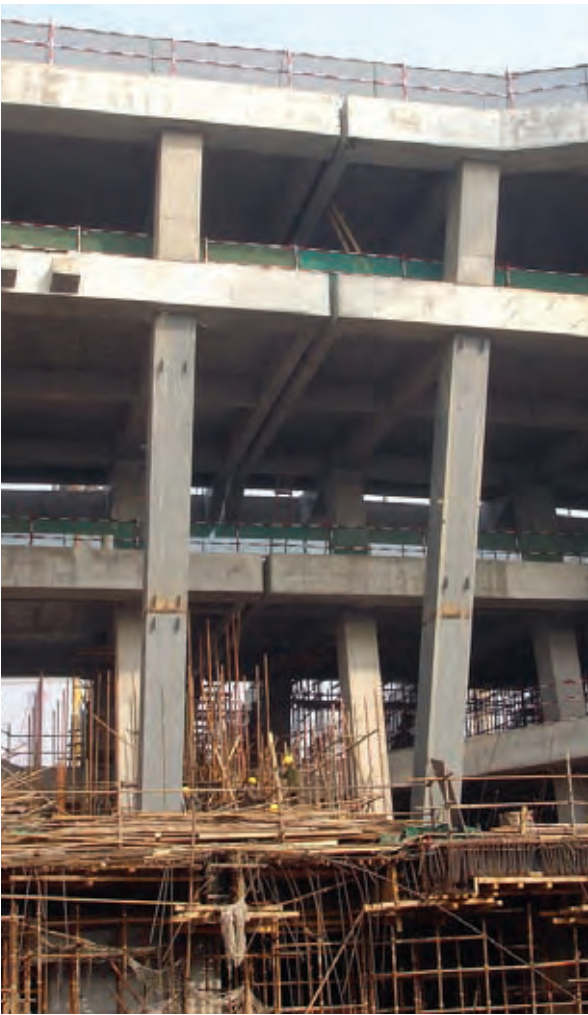
1. Movement/seismic joint between segments of the bowl structure.
