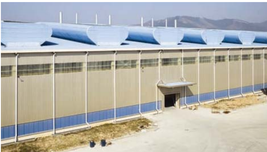
27. Roof ventilation on completed building.
