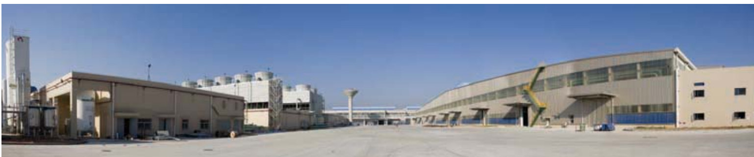
22. Zone 9 utilities on the left, and Zone 6, package and shipping, on the right.
