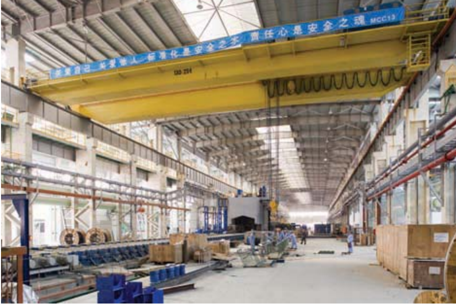
8. Rolling table and overhead crane in Zone 2 hot rolling mill.
