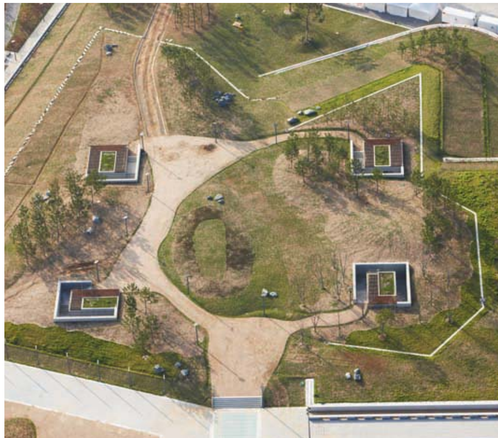
20. Landscaping above the underground parking garage, showing bulkhead access.
