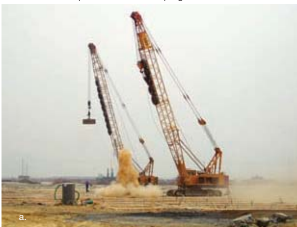
23. Ground improvement works in progress.
