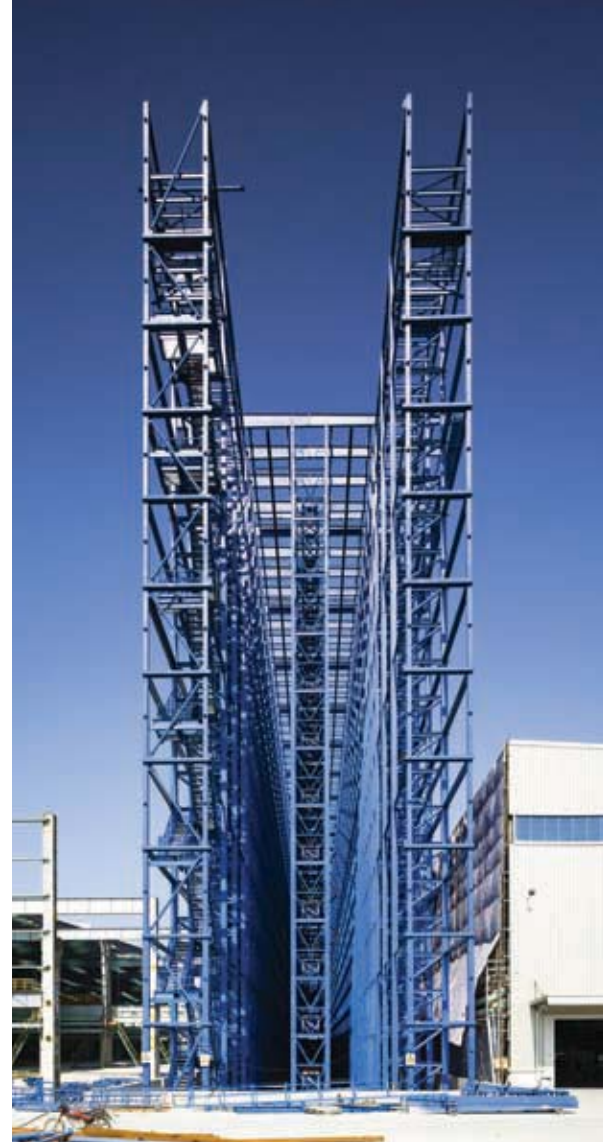
18. The 45m tall high bay store under construction.
