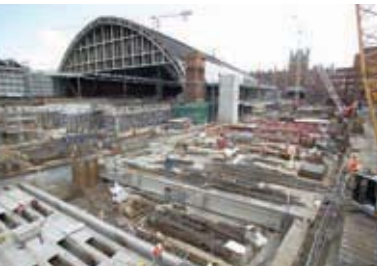
7. Roofing the box opposite St Pancras platform extension, October 2004.
