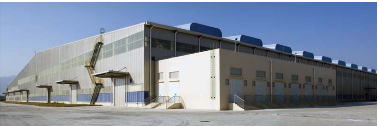
13. Transformer rooms are generally outside the main production facilities.
