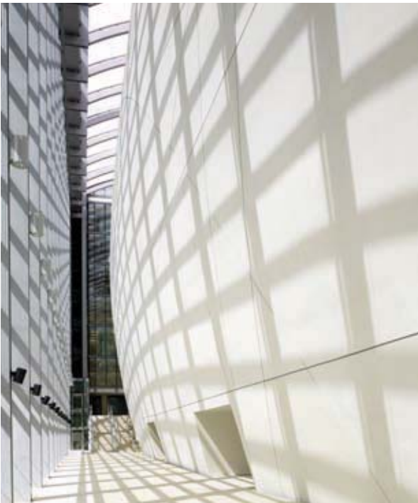
5. Internal view of the completed cocoon.
