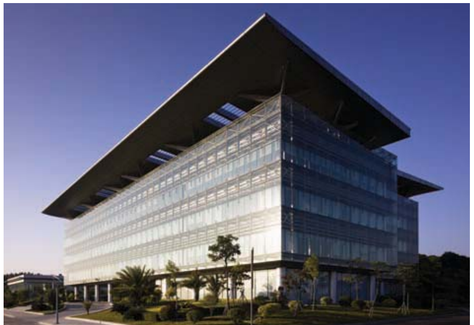
30. Rear elevation of the office building.
