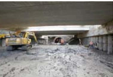
8. Excavating main Thameslink station area, October 2004.
