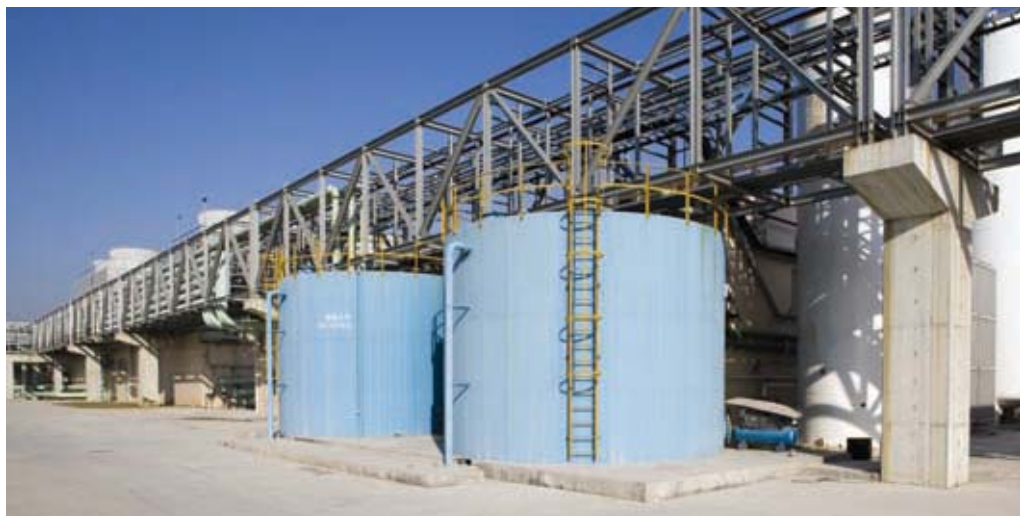
29. Pipe bridge for supporting services pipeworks connected to the factory buildings.
