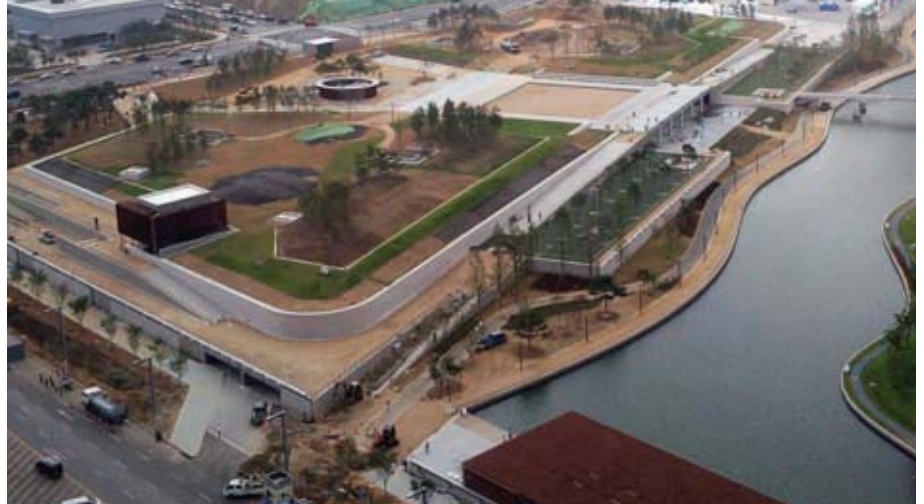
17. Aerial view of underground parking garage.
