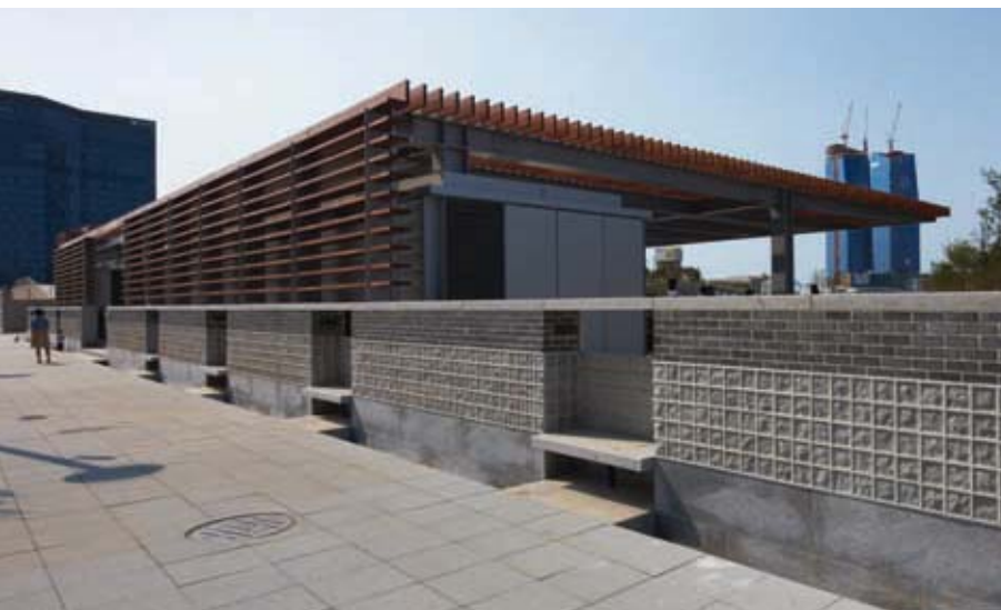
24. Exterior of Boathouse West.
