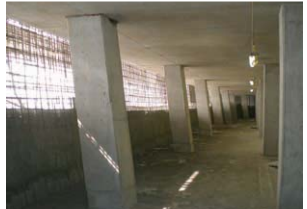
21. Temporary columns with spraying of the concrete shell in progress.
