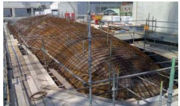
15. Cocoon reinforcement.
