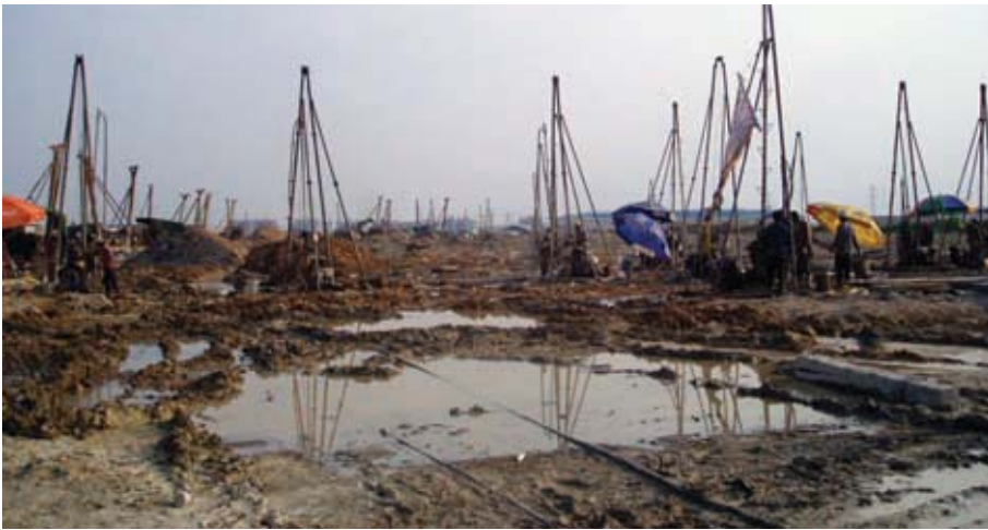
19. Drilling rigs as far as the eye can see.
