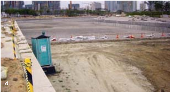
15. Canal bed construction: Above (a) Prehydrated GCL laid down on existing reclamation fill; (b) Soil layer added for soft protection of liner; (c) Recycled plastic honeycell layer filled with crushed stone to provide adequate protection cover; (d) Phased operations along canal; Below (e) Finished product.
