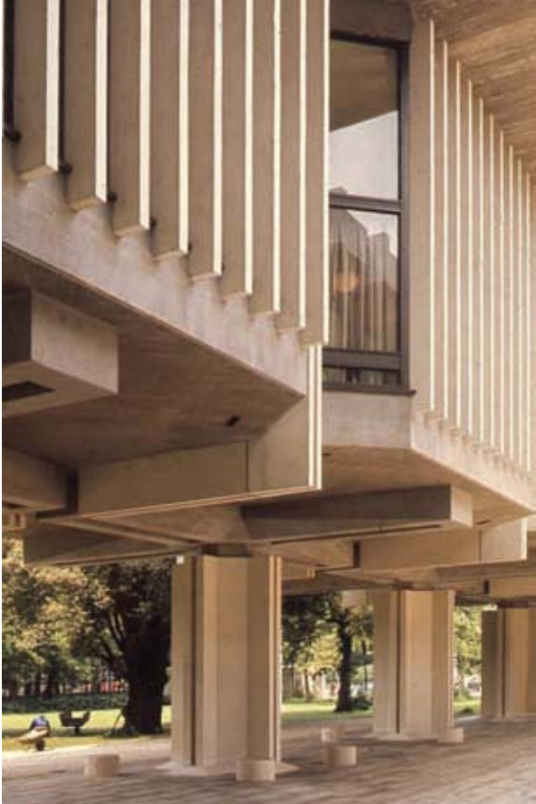
6. Detail of vertical solar shading within courtyard.
