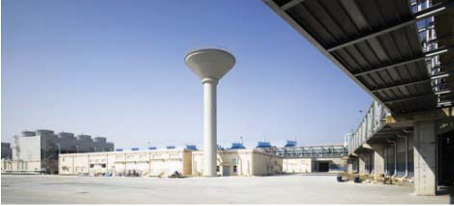
31. Water storage tower and utilities building.
