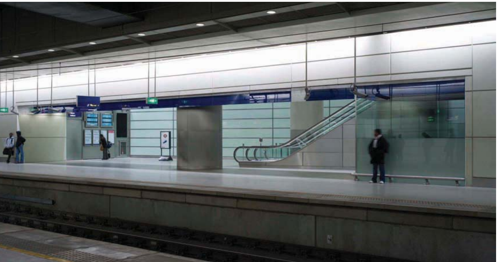
12. Glazed wall panelling, stainless steel clad bases to the concrete columns and terrazzo flooring feature throughout the public areas, including the platforms.
