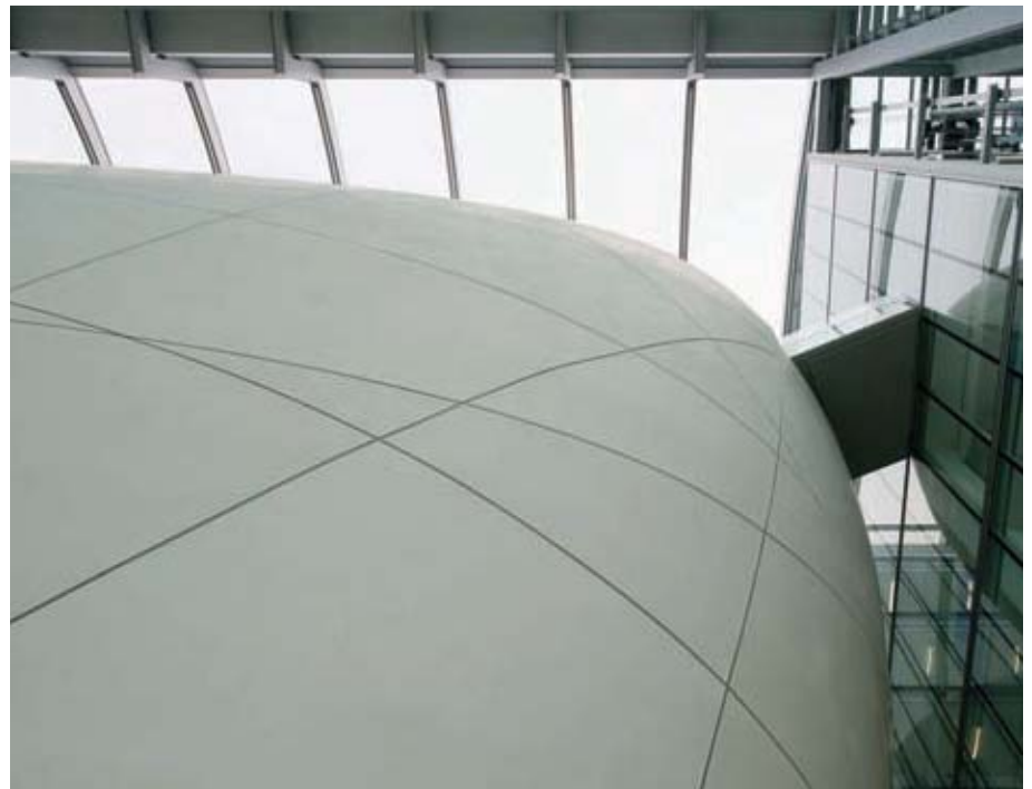
7. Cocoon end showing polished plaster finish with expansion joints.
