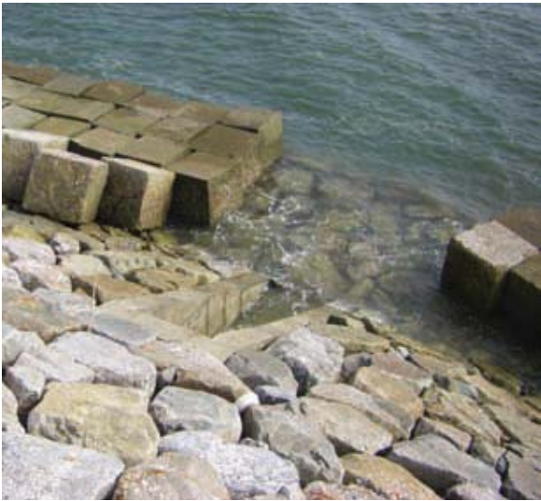
10. Sea wall intake after construction.
