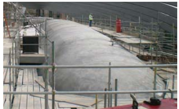
16. Completed concrete surface.
