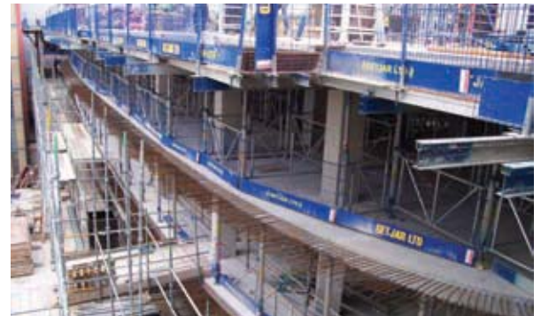
19. Cocoon slabs with protruding starter bars.
