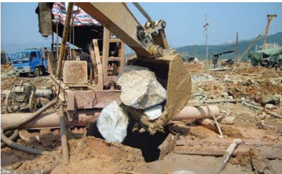
20. Cavity remedial works.
