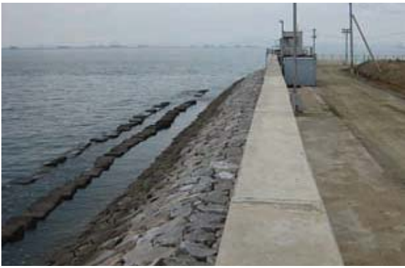
9. Sea wall at intake location prior to construction.
