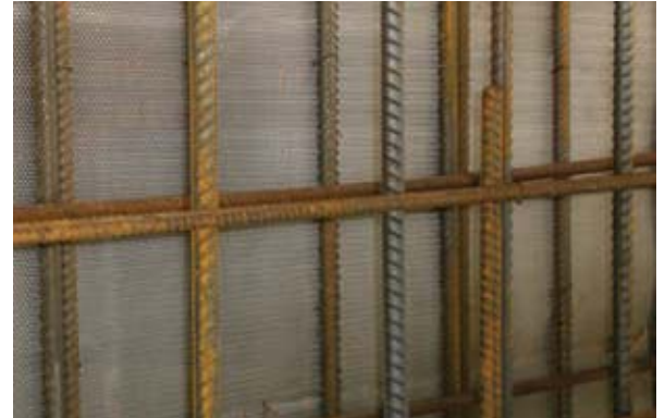
20. Expanded metal mesh connected to the inner shell reinforcement.
