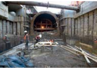
6. Construction at the south end of the box, October 2004.
