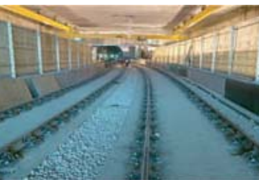
9. Track laid in main station area, March 2005.
