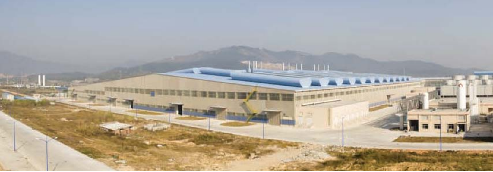
1. Overview of the flat rolled product facility designed and project managed by Arup.
