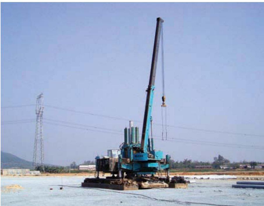
21. PHC piles for factory foundations.
