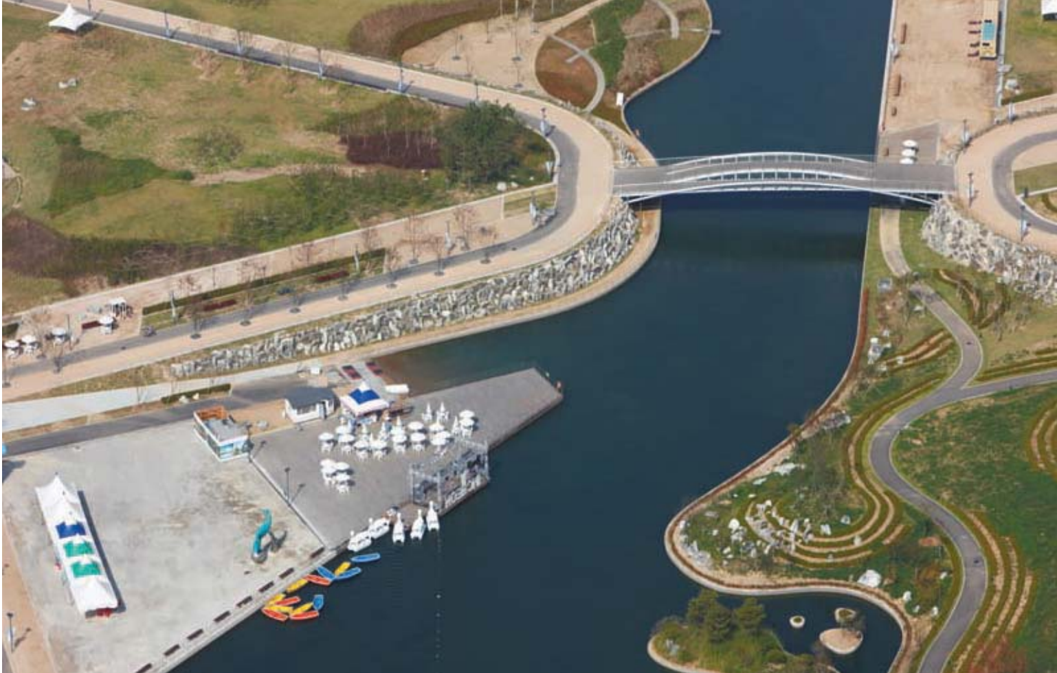
26. Park Path Bridge in context, with part of the ecology centre at the bottom left.
