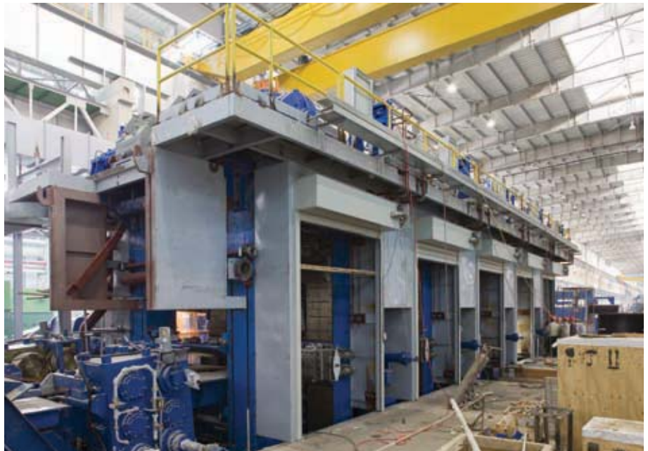
16. Installation of the five-stand hot rolling mill.
