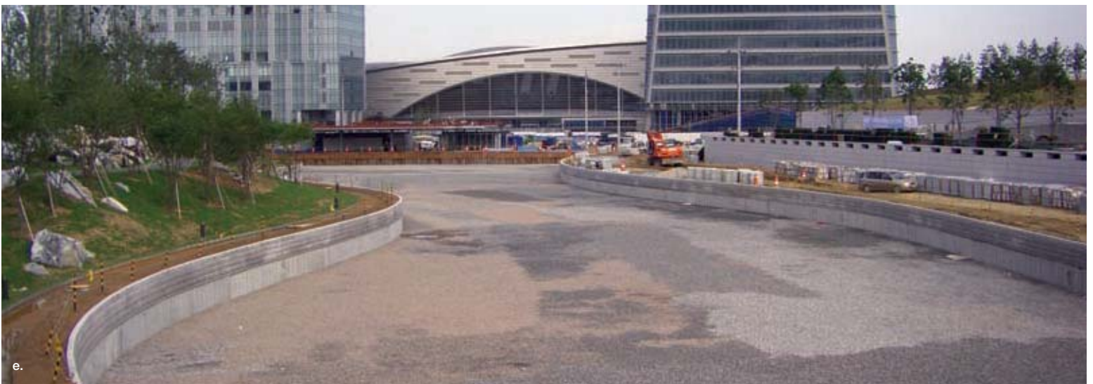
15. Canal bed construction: Above (a) Prehydrated GCL laid down on existing reclamation fill; (b) Soil layer added for soft protection of liner; (c) Recycled plastic honeycell layer filled with crushed stone to provide adequate protection cover; (d) Phased operations along canal; Below (e) Finished product.
