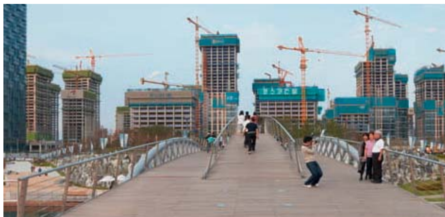
27. The deck surface of Park Path Bridge, with blocks D22 & 23 in the background.
