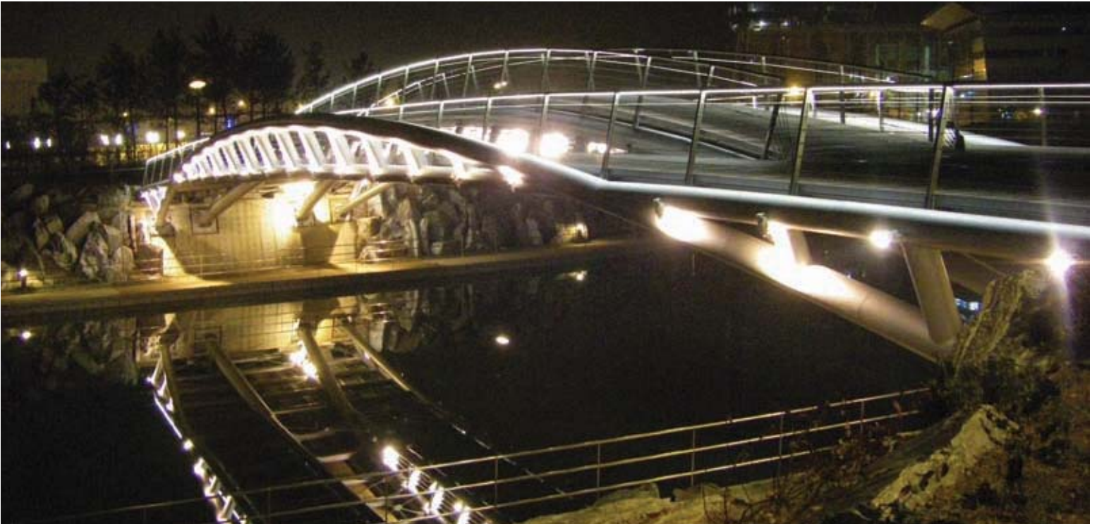
22. Park Path Bridge at night, showing feature lighting (see pp14-15).
