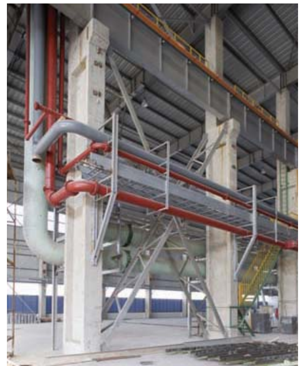
4. Typical factory building showing concrete columns supporting the structural steelwork.
