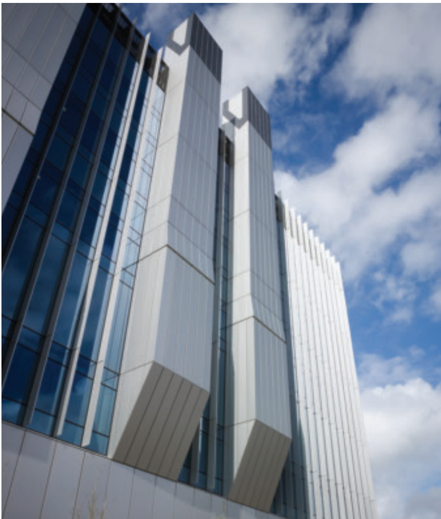
4. Harlequin 1 building at BSKyB campus.
