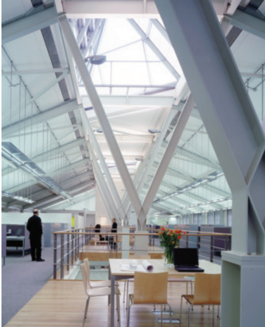
1. The Arup Campus, Solihull, West Midlands (see p8).
