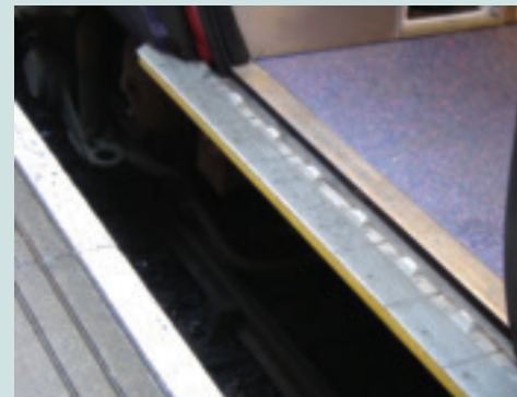
3. Larger gap at north end of the platform.
