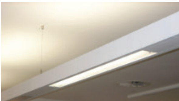
3. The illuminance was set to 300 lux which was achieved using 50% up light and 50% down light.
