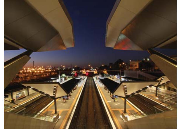
22. View from new concourse overbridge onto platforms, with existing heritage listed station facility in the background.
