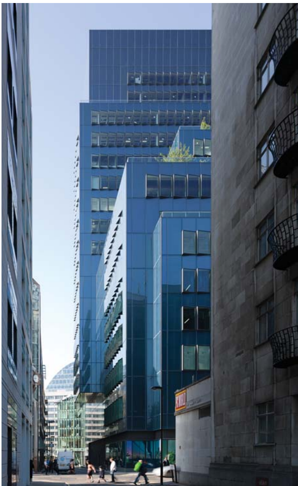
9. Looking south along Finsbury Street.
