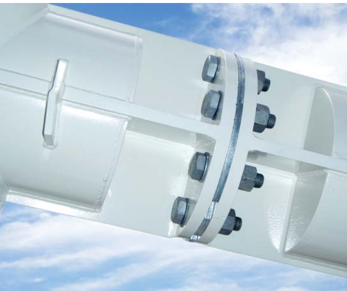
16. Bolted splice connection.
