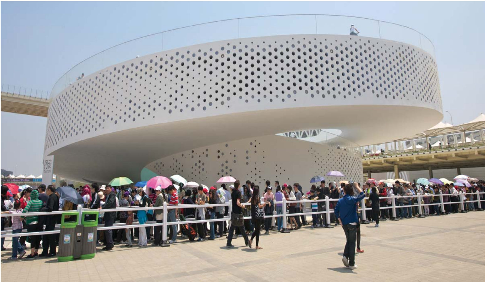
5. Perforations on façade.
