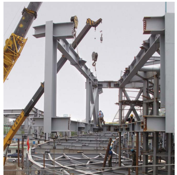
17. November 2009: Steelwork in progress.
