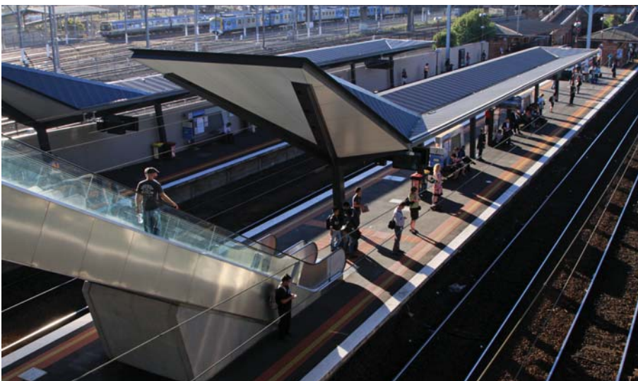
8. Finished station from the concourse level above platform 4.
