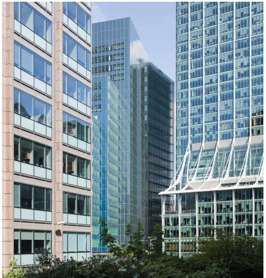
10. The south-west corner of Ropemaker Place.
