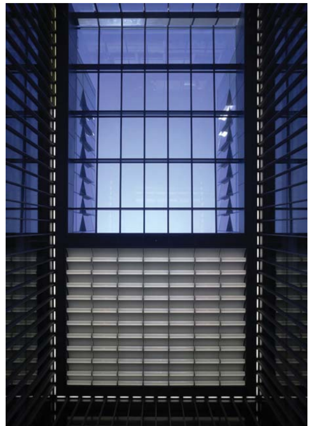
14. Glazed atrium roof.
