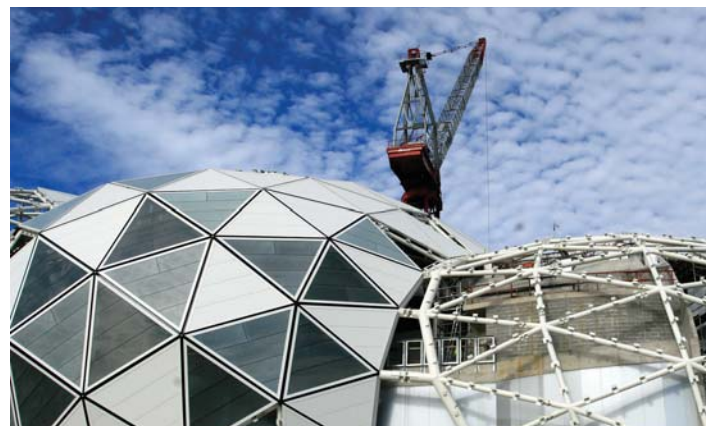
23. Installation of façade panels.
