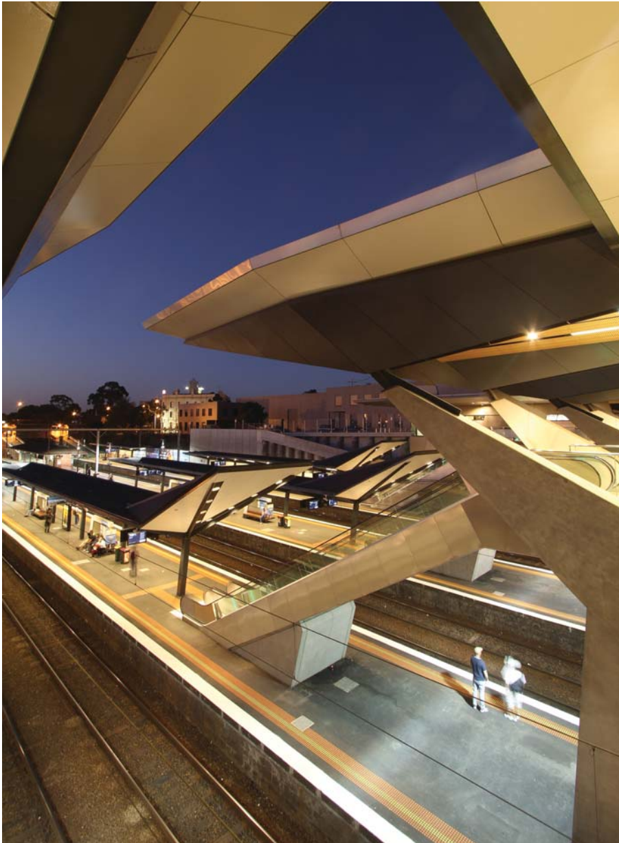
1. The finished station from the concourse level above platform 6.
