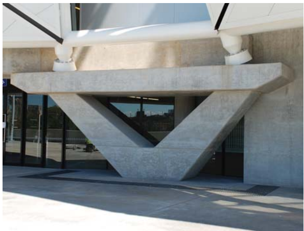
20. V-column supporting vertical loads.
