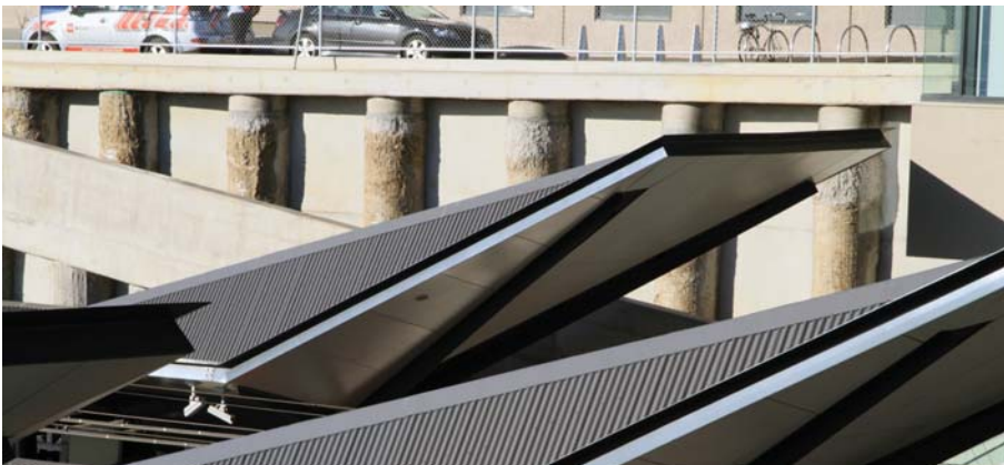
7. Finished platform canopy roofs with 6m high retaining wall and access road in the background.
