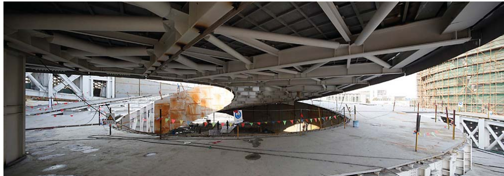
22. December 2009: secondary steelwork finishing, surfacing, and railing.
