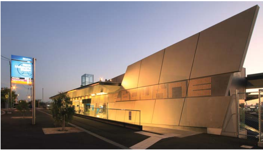
2. The new station entrance and station building from the forecourt on top of the embankment.
