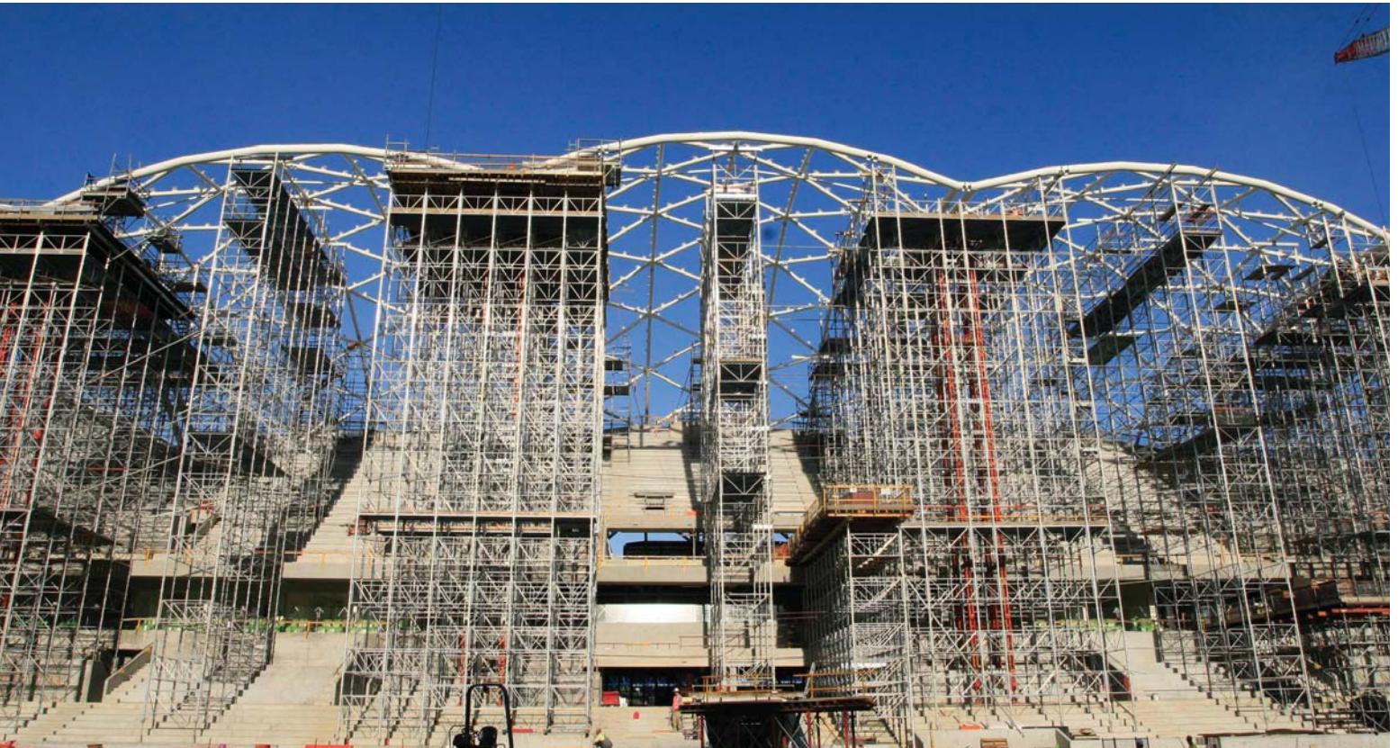
11. Steel roof under construction.
