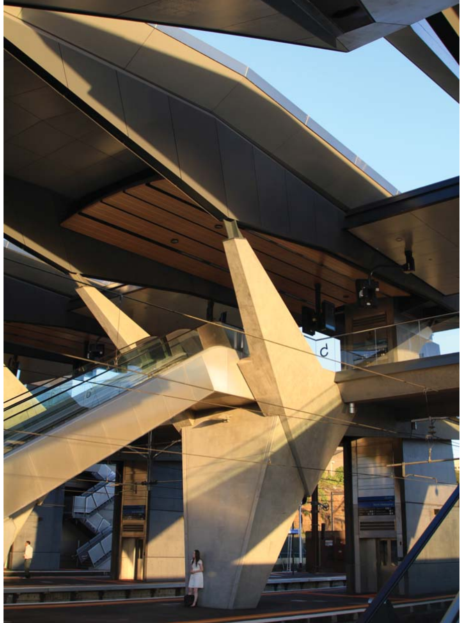
12. The main impact-resistant support pier from platform level.
