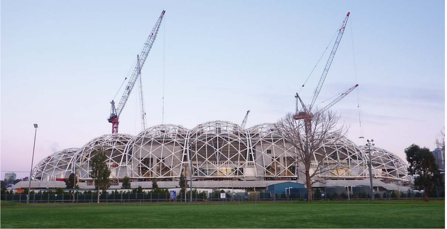
12. Steel roof structure in place.
