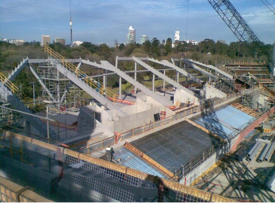
10. Steel rakers being constructed.
