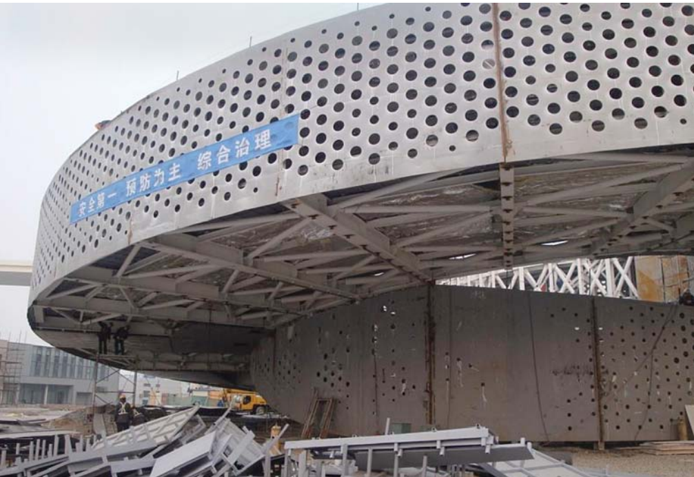
23. December-January 2010: Cantilever unpropping.
