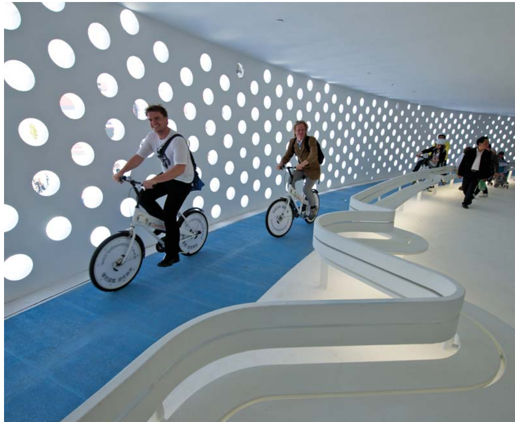
11. Perforations in the structure allow light and ventilation to penetrate the building.
