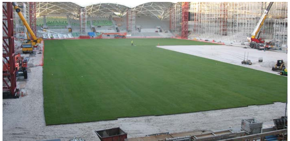
27. Playing surface being installed, April 2010.
