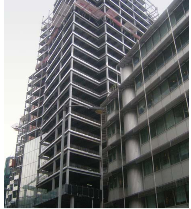
32. Steel frame nearing completion, and façade commenced.
