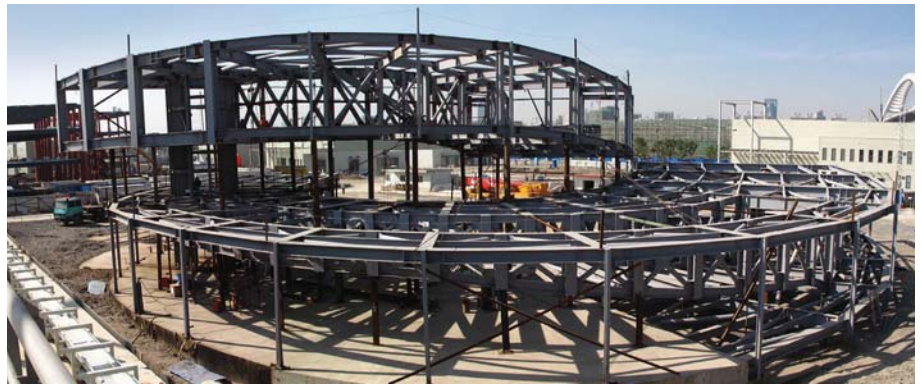
21. November 2009: first frames erected.
