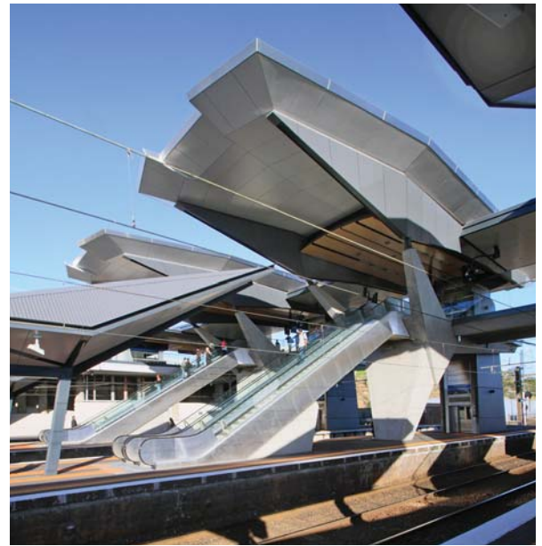
20. Completed concourse structure from platform level.
