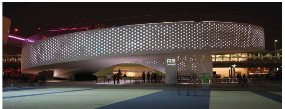
12. Exterior view at night showing the open nature of the building.
