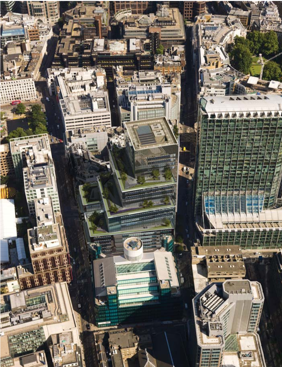
3. Ropemaker Place in its urban context, showing the overall form of interlocking cubic volumes.
