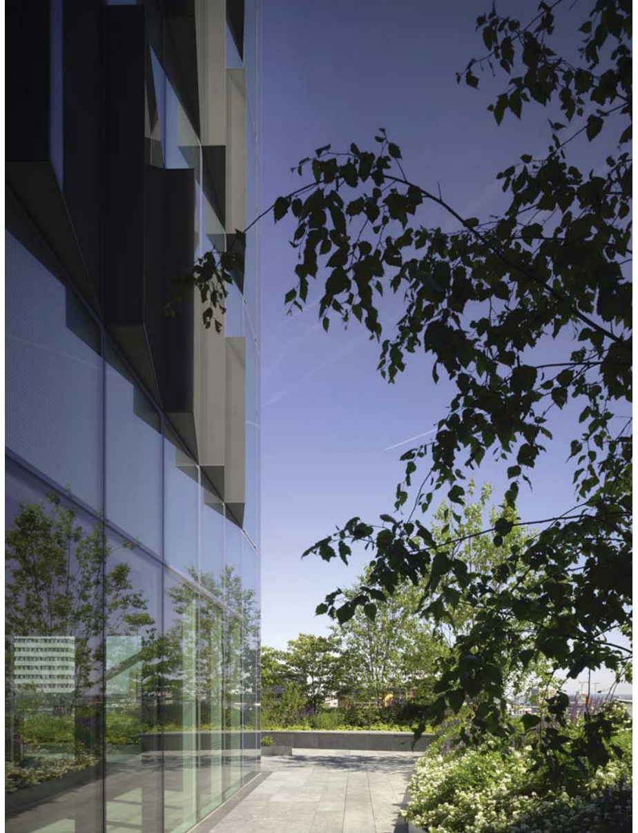
16. Typical planting on one of the roof terraces.
