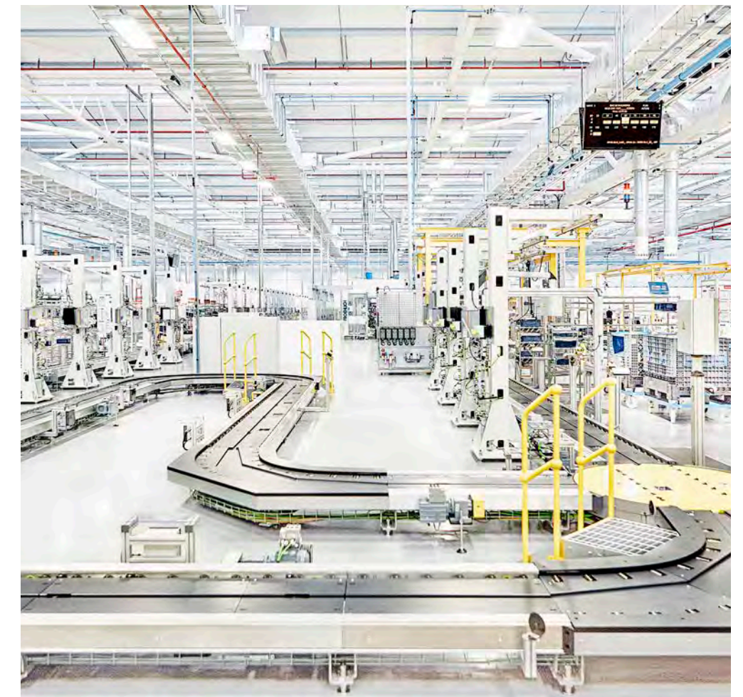
6: Arup, in conjunction with the client, developed an overall facility layout that focused on efficiency and future building flexibility
