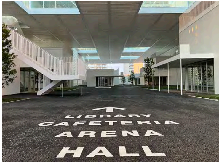
1: A key design feature of the new Nagoya Zokei University is a central 'art street' that passes through the building
