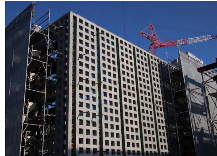
13: Strain gauges were attached to the steel plates and demonstrated that stresses caused by concrete shrinkage would not affect the bearing capacity
