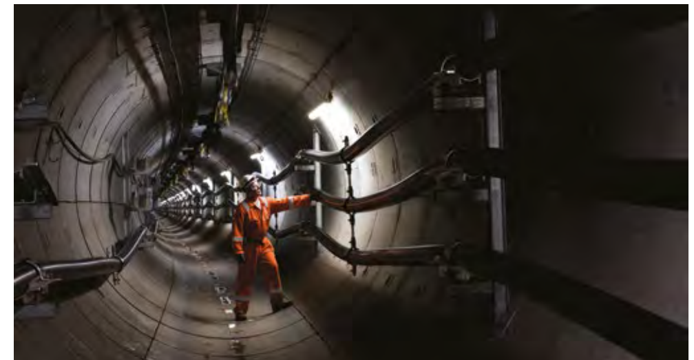
▼ LONDON POWER TUNNELS London, UK
