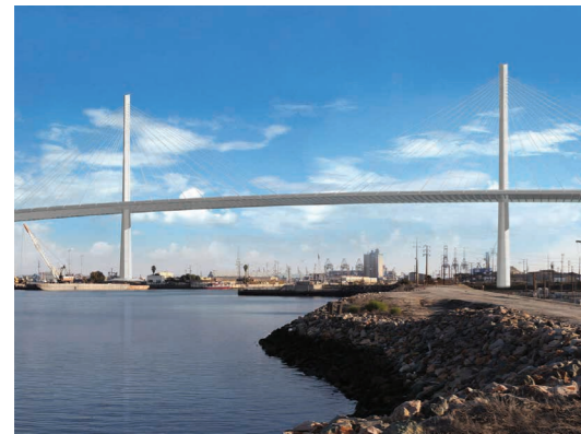
Gerald Desmond Bridge, California, USA
