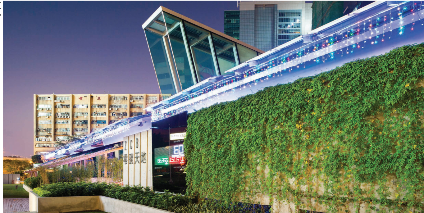
CIC Zero Carbon Building, Hong Kong
