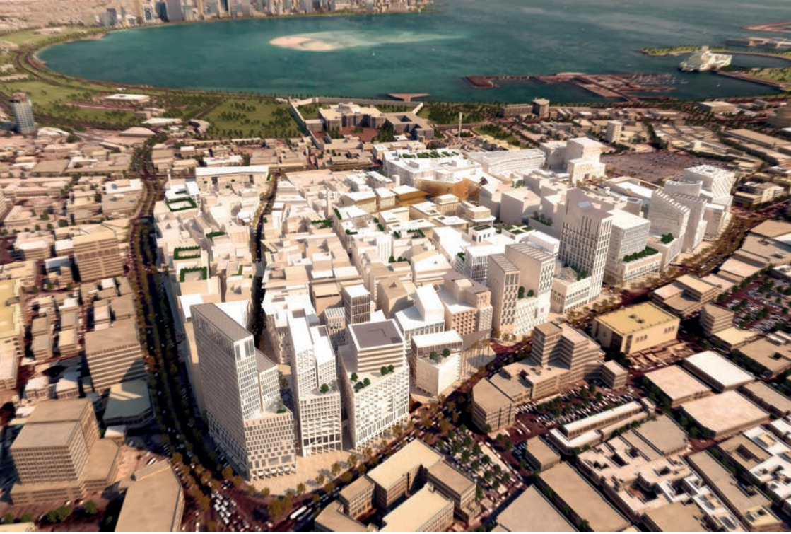
▲ Msheireb Downtown Doha in Qatar
