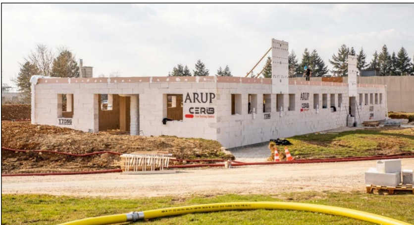
Figure 68: Large compartment experiment building
