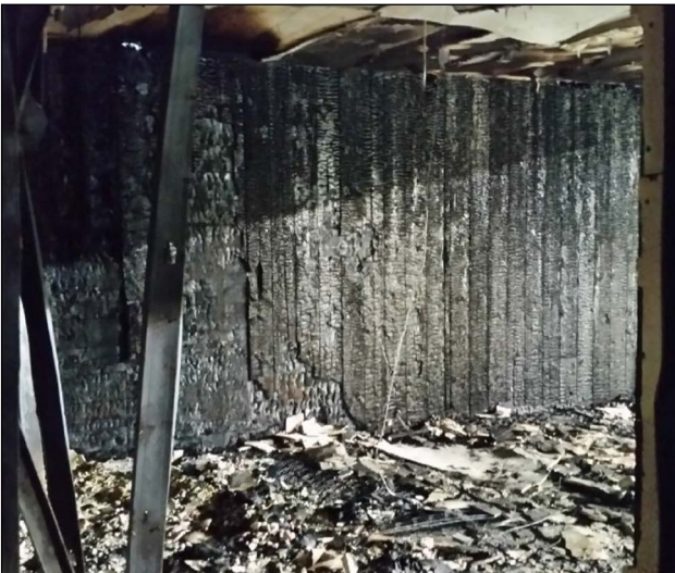
Figure 43: USFS-ICC – Test 3 – Post-test photo
