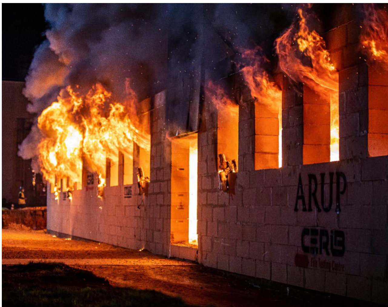
Figure 2: CodeRed - Experiment 1 with a fully exposed CLT ceiling
