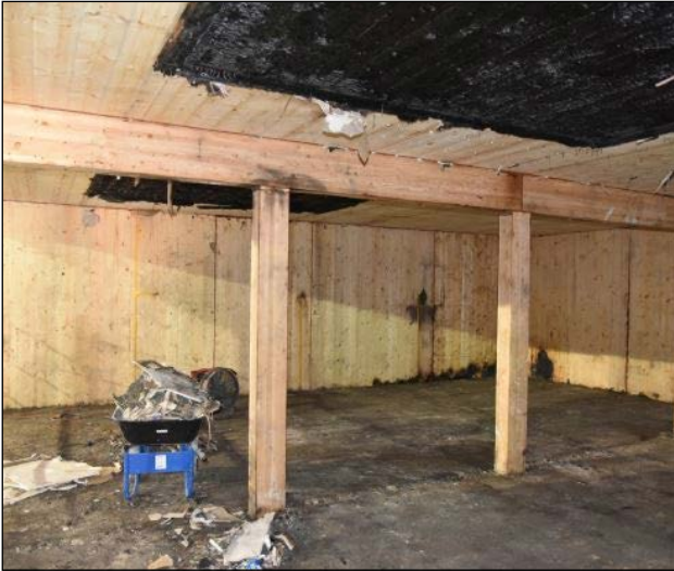
Figure 41: USFS-ICC – Test 2 – Post-test photo – 30% exposed ceiling
