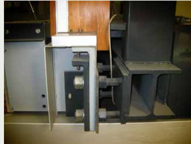
Fig 5: Lower spandrel unit
