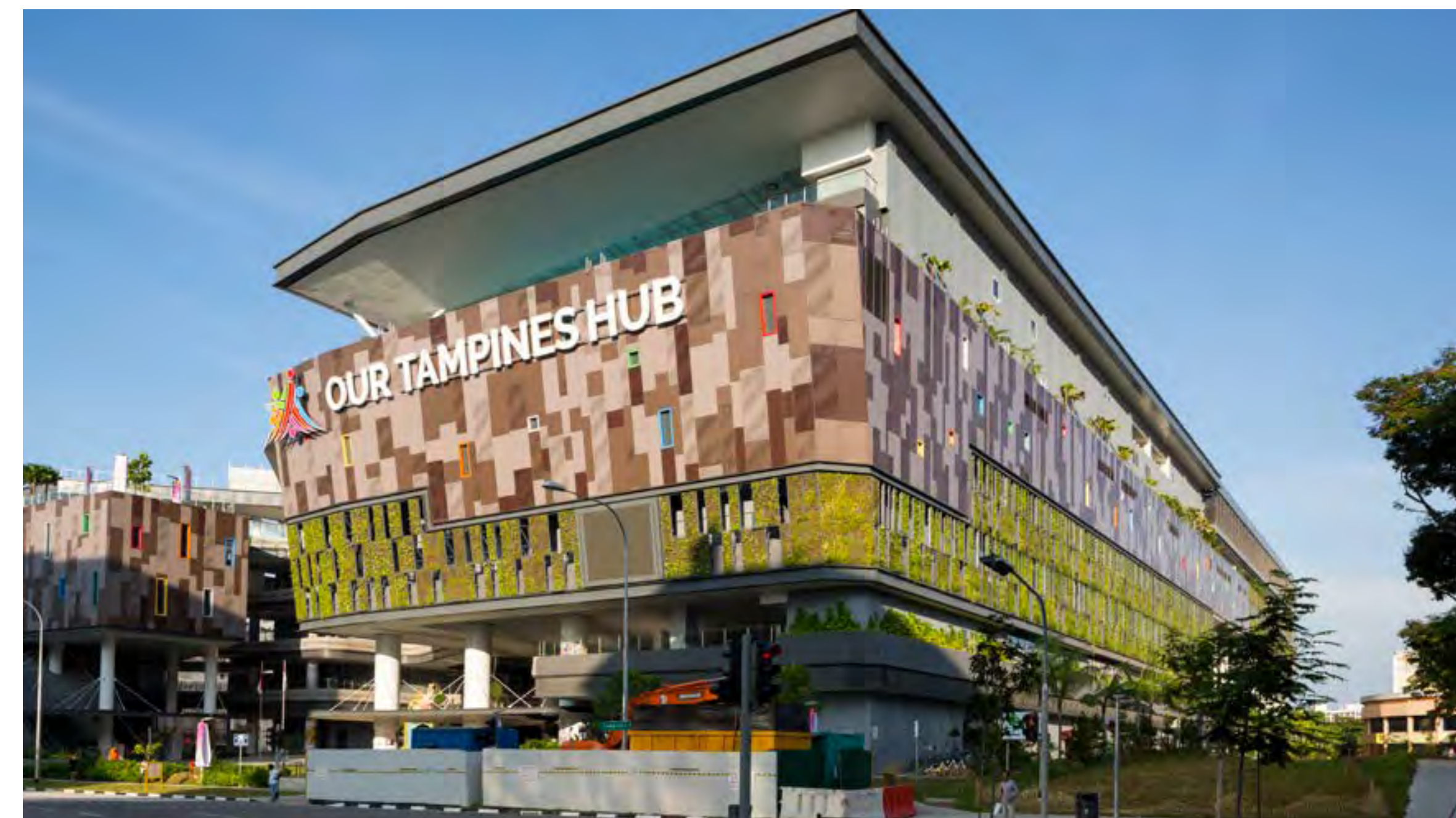
Our Tampines Hub (sports facilities)
