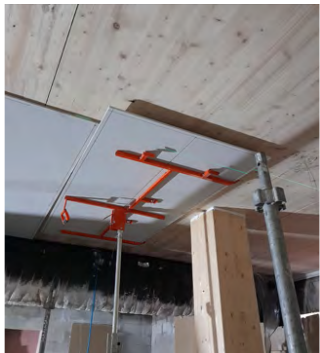
Figure 10. Installation of board protection to the CLT ceiling.
