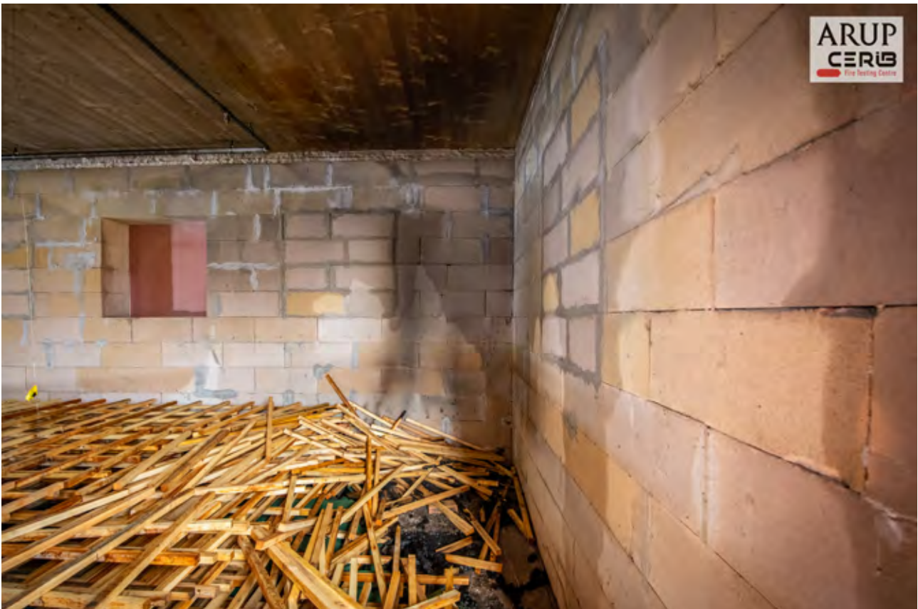
Figure 8. Ignition of the wood crib at the corner of the building, and activation of suppression system.
