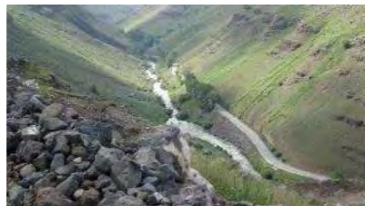
Adjaristqali (Shuakhevi) hydropower project (180 MW), Georgia
