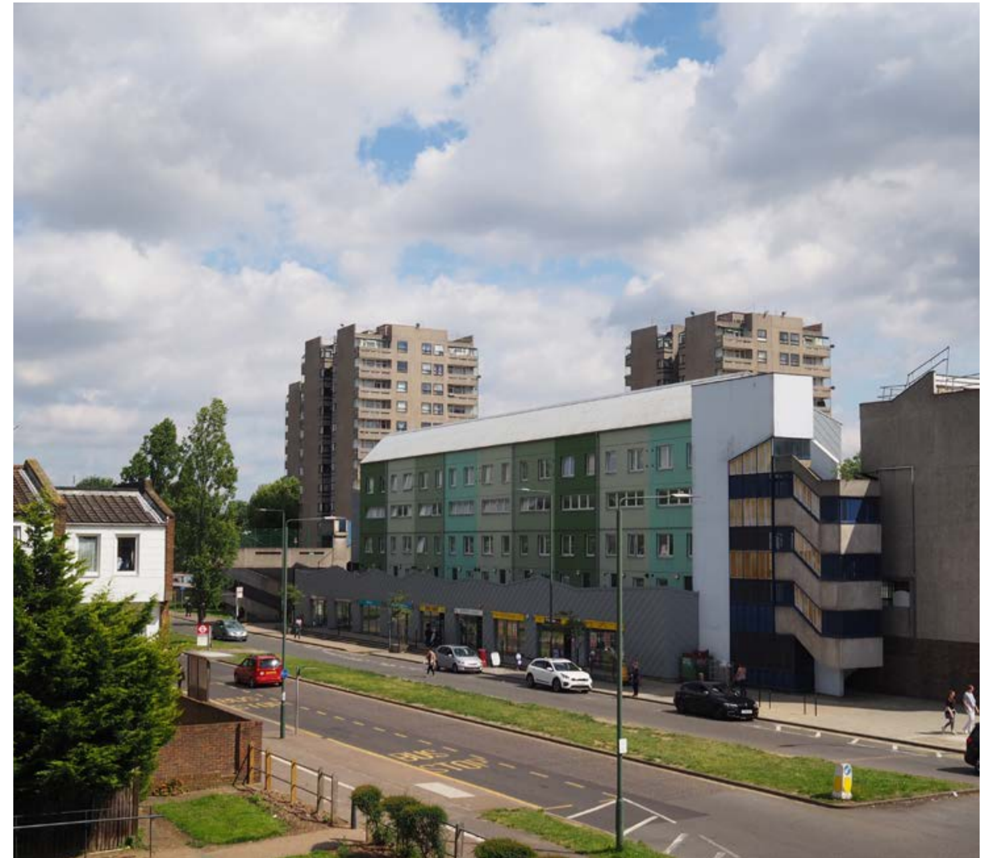
A view over Yarnton Way to Jacob, Masham, and Clydesdale House on the Thamesmead estate.
