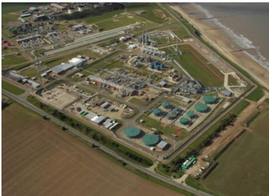
Figure 56: Bacton Gas Terminal (© BBL Company)
