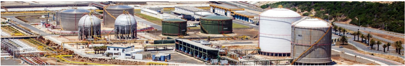
Figure 82: Port of Sines Petrochemical Terminal. Source: (Port de Sines, n.d.).
