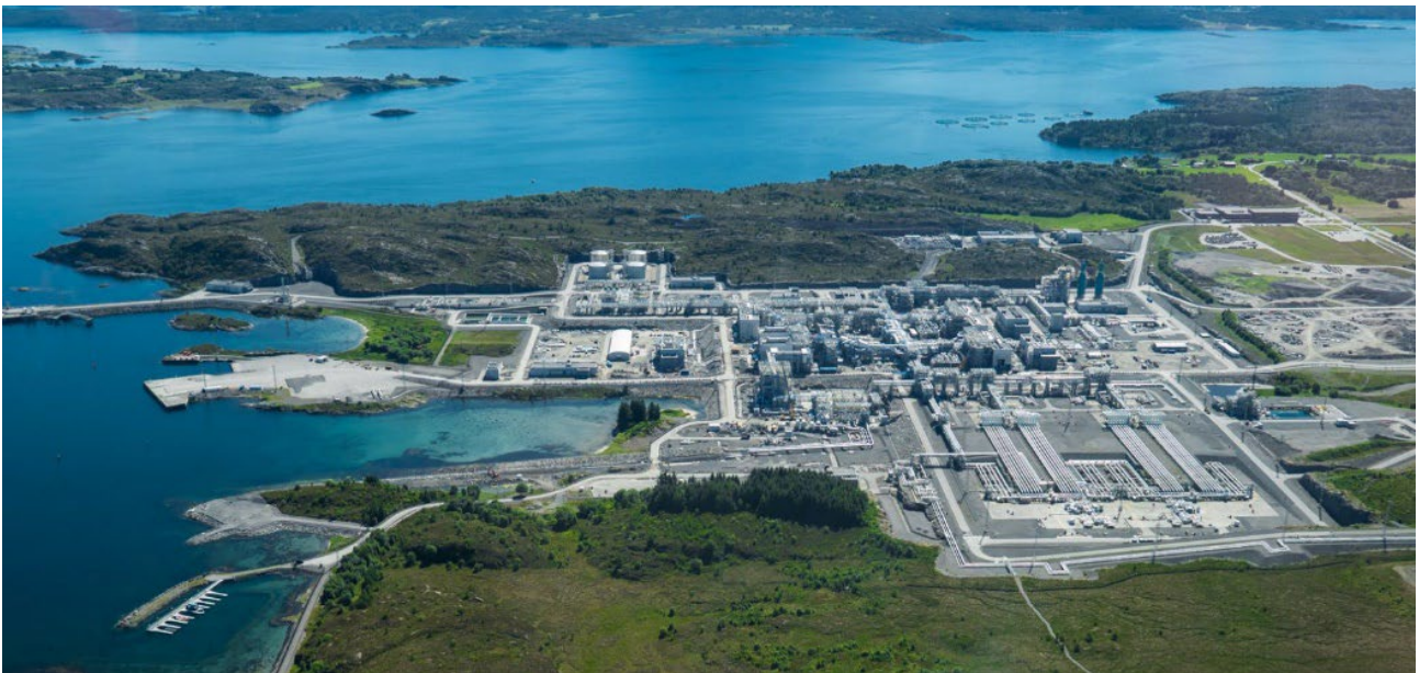
Figure 60: Nyhamna Process Plant (© Gassco)
