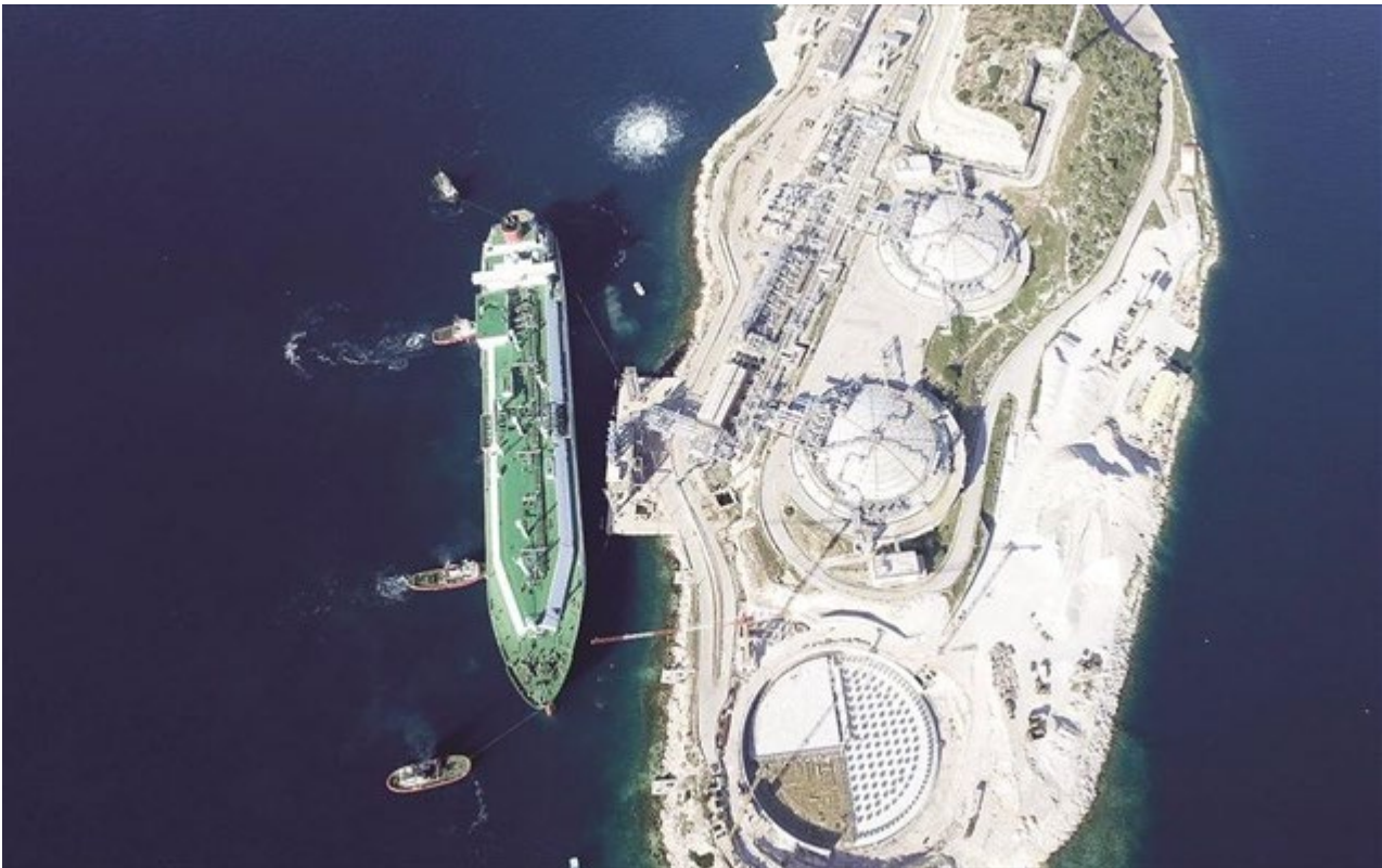
Figure 81: Revithoussa LNG terminal. Source: (DESFA, n.d.).
