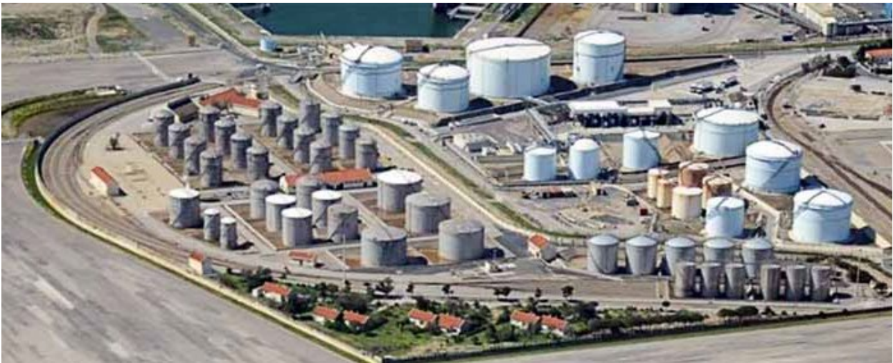
Figure 80: FOSELEV terminal. Source: (Port La Nouvelle, n.d.).
