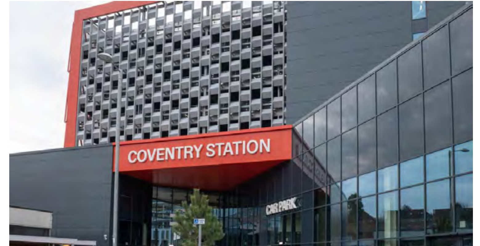
Coventry Station redevelopment © Rail Business UK
