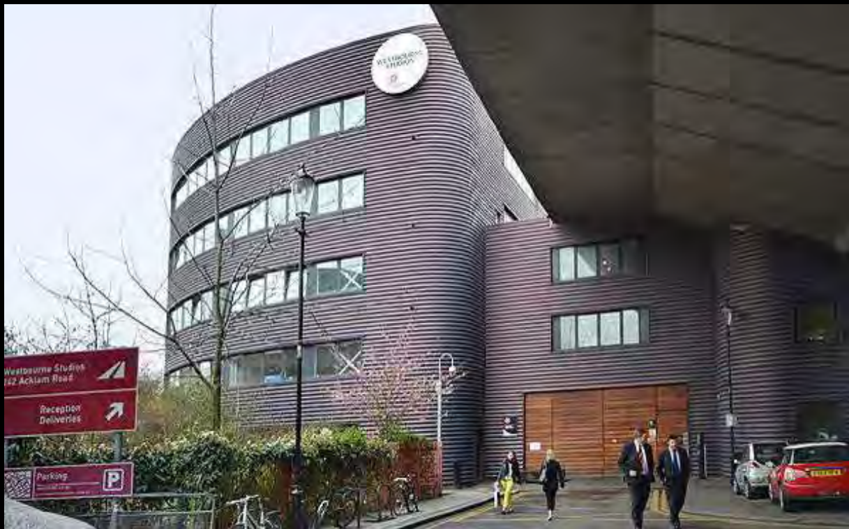
Above: Two medium-rise blocks protrude either side of the carriageway. Below: Between these blocks an elegant multi-functional space forms the focal point, with the exposed concrete under-side of the viaduct structure forming a distinctive ceiling
