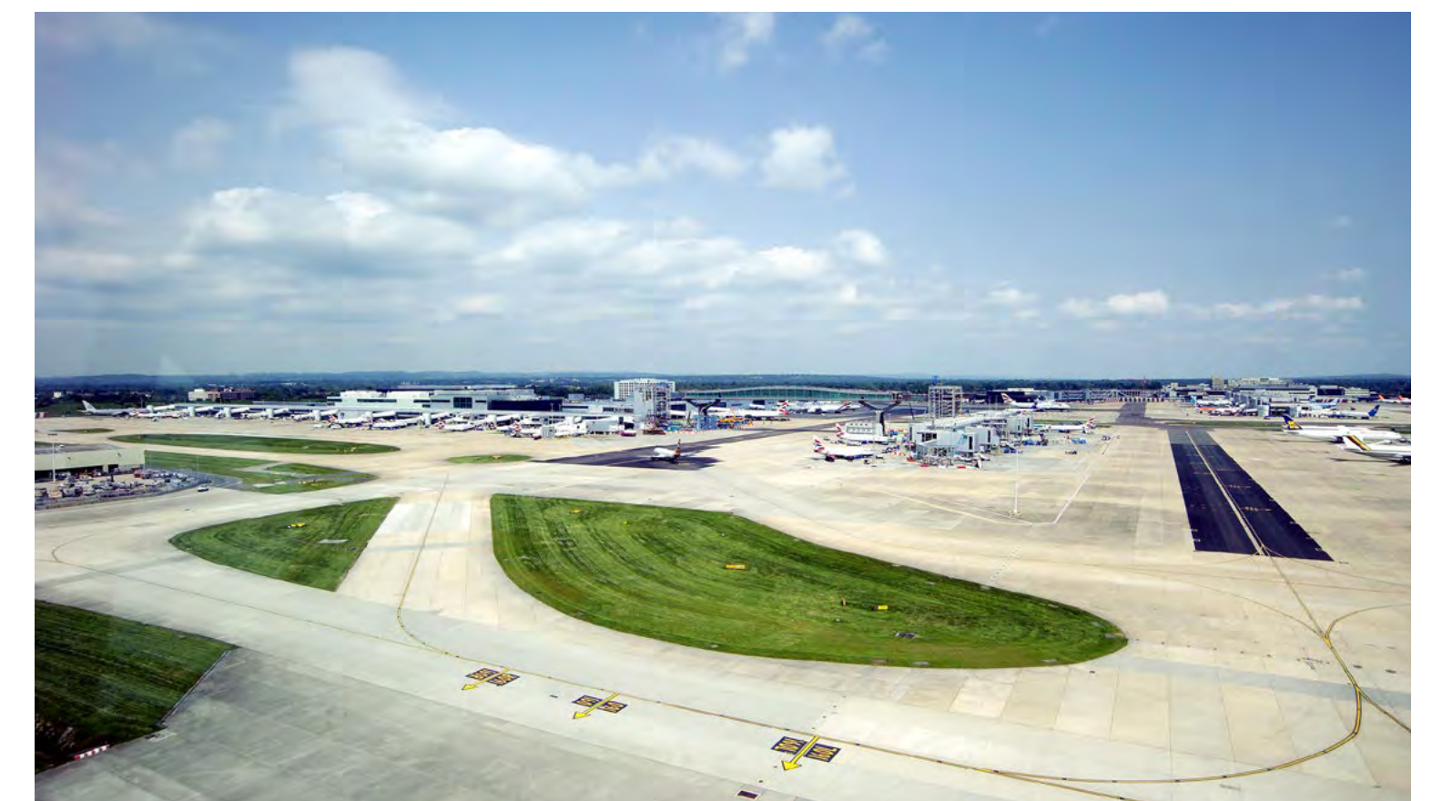
London Gatwick Airport Bridge, UK
