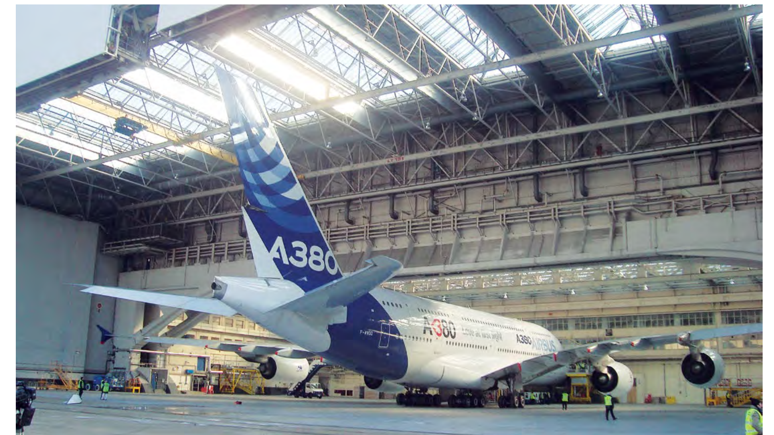
A380 Hangar, London Heathrow Airport, UK
