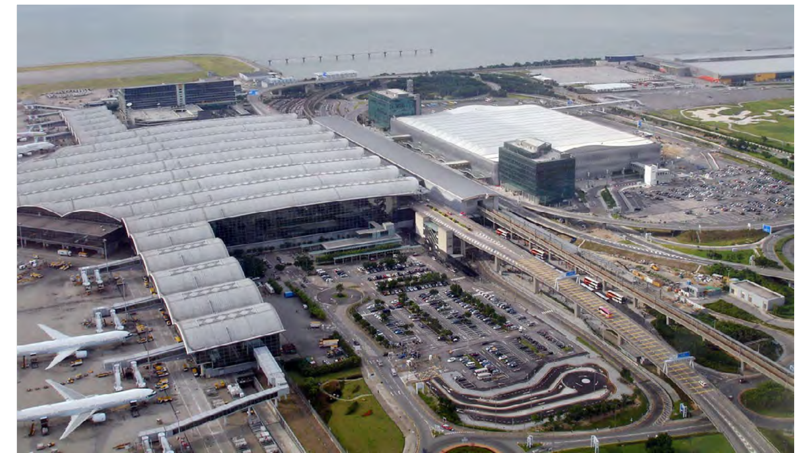
Sky Plaza, Terminal 2, Hong Kong International Airport
